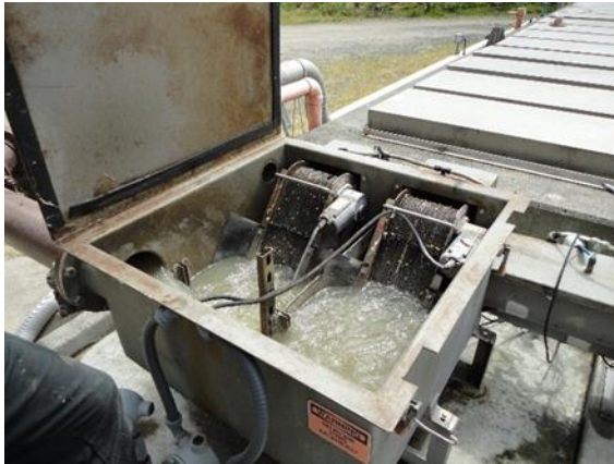
Figure 5. Picture of the Headworks of the MBR Plant Prior to Upgrade
