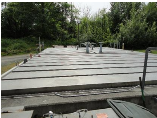
Figure 6. Picture of the MBR Basins
