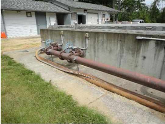
Figure 7. Picture of Pipe from Anoxic Basin to Pre-Air Basin (components of MBR)
