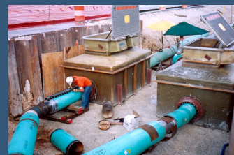
Hydrant piping vaults
