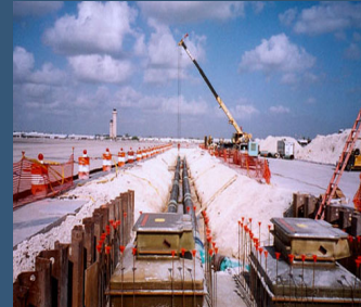
Installation of AHS piping and vaults
