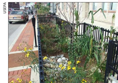
Figure 10. Bioretention planter boxes in Lansing capture and treat much of the stormwater from roads and sidewalks.
