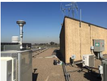
Figure 10.2 San Ysidro – Pictures (Directional) from the Roof
