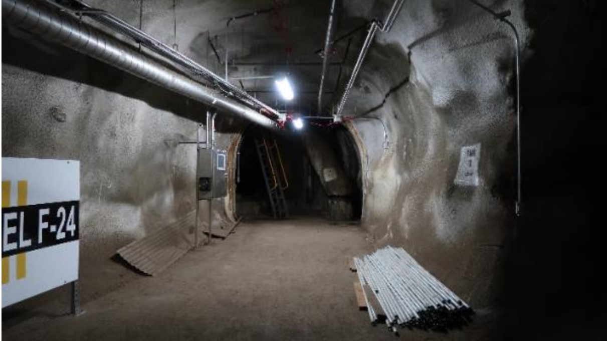
Looking down tunnel center below Tanks 1-2 Tank Gallery with no contractor equipment. Galleries are 200 feet apart
