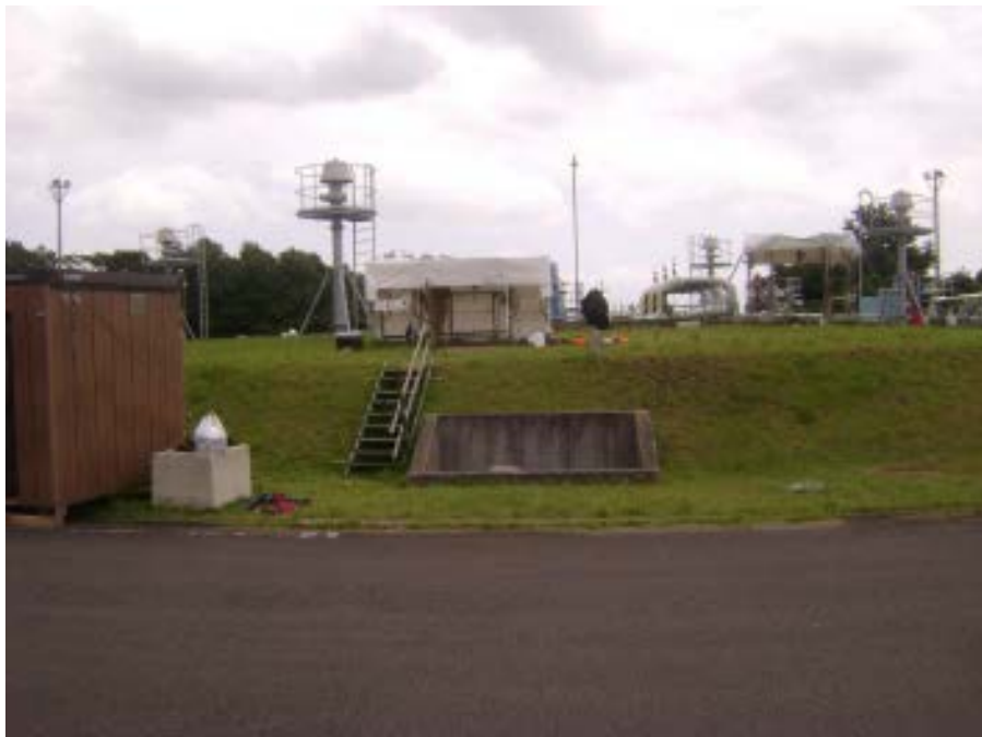
Exterior of Tank Y-8 – West Elevation
