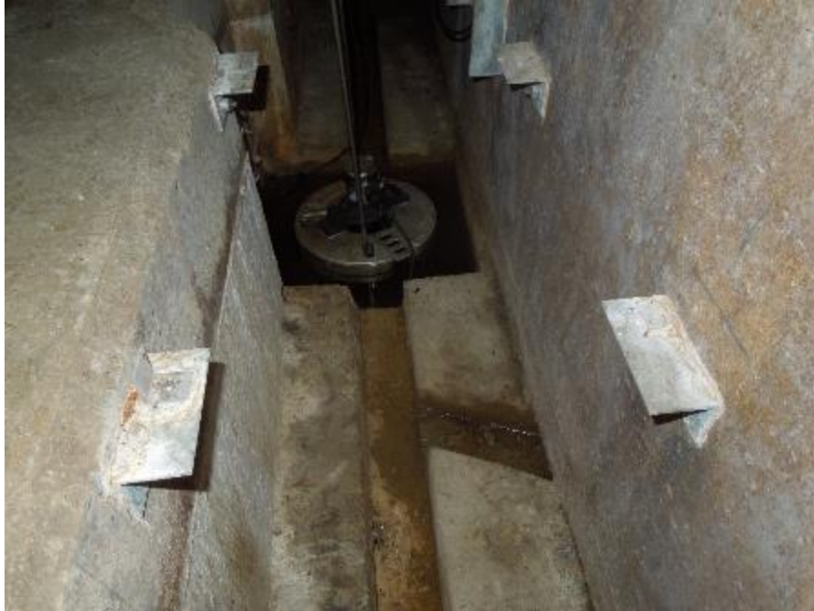
Oil Leak Detection Alarm in Gallery Space, Drainage Slots Below Floor Note: Floor grating removed for photo. Drainage slots exit to gallery trough.
