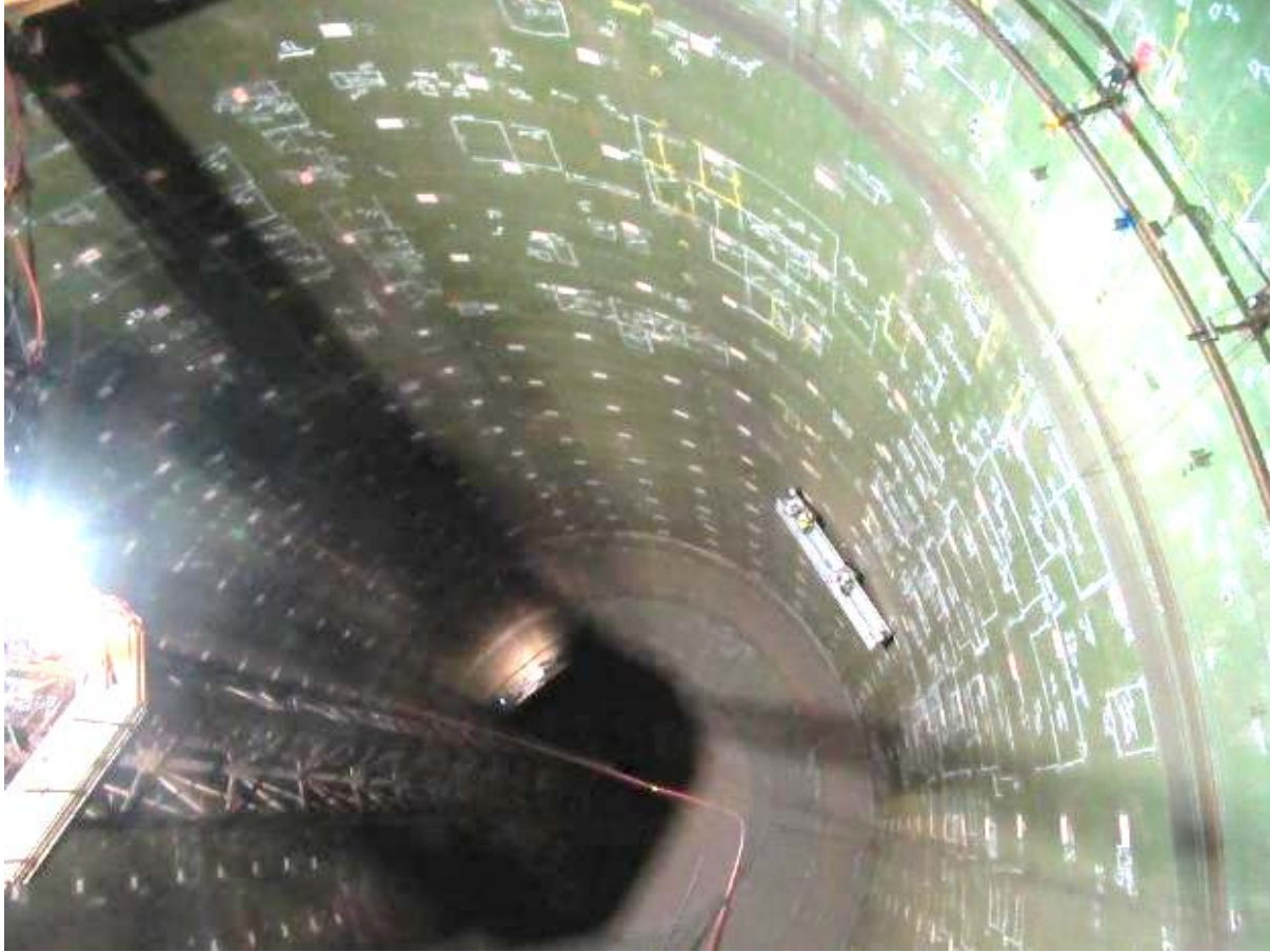
Personnel Platform utilizing Monorail System at Top Right.
