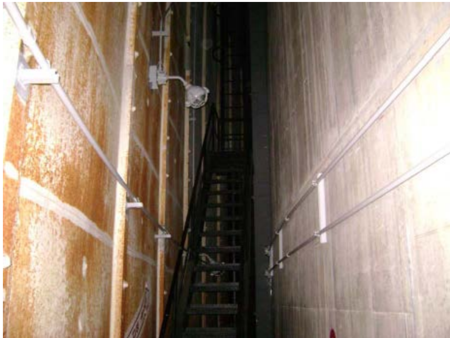
Ladder and Stair Access into Gallery Space (Typical of 4) (Note: Original tank barrel is on the left side; tank shell is on right)
