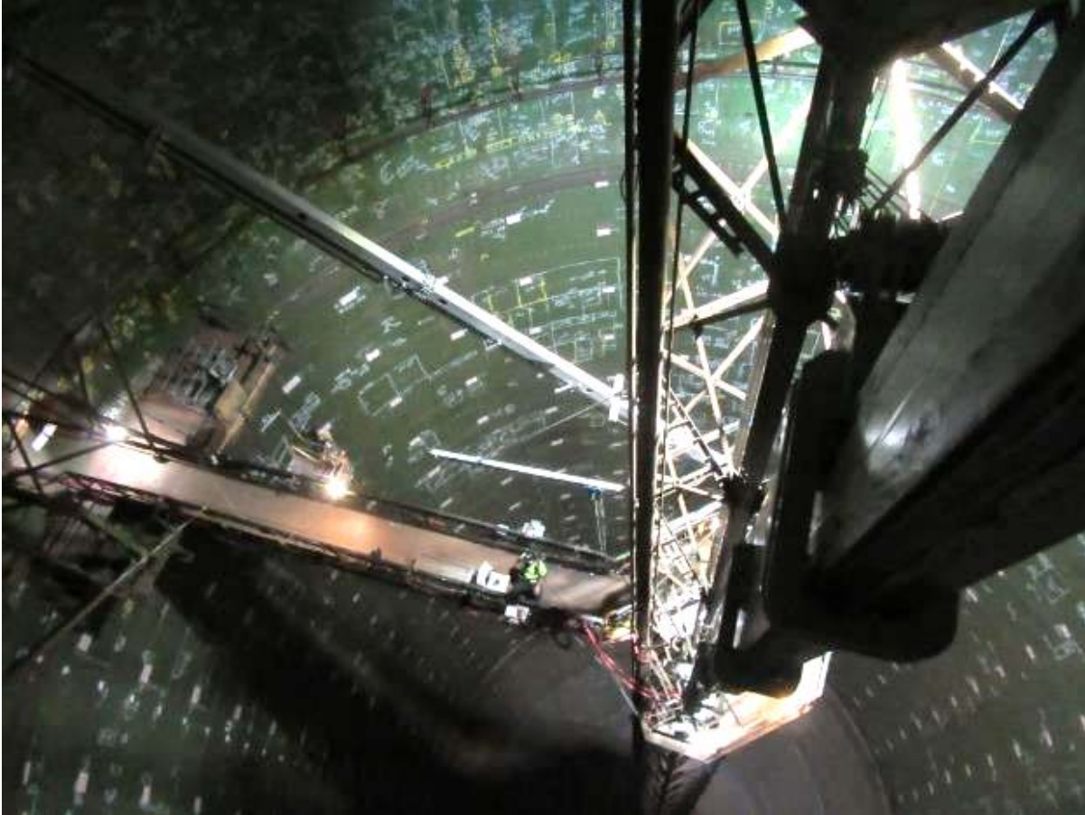
Catwalk and Small Access Platform from Tank Manhole. Note boom on right hand side. Photo was taken from basket on boom.
