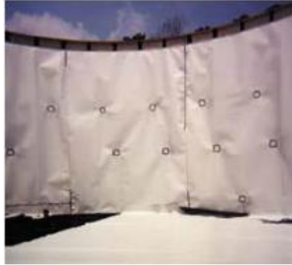
Bolted HDPE Liner inside Tank – GFR (19)
