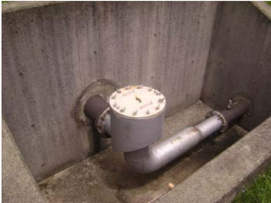
Fire (Foam) Injection Port (Typical of 4)
