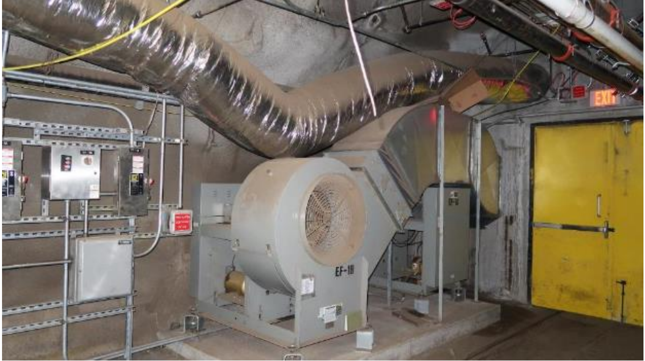
Existing Upper Tunnel Exhaust Fan Note temporary construction venting duct above fan
