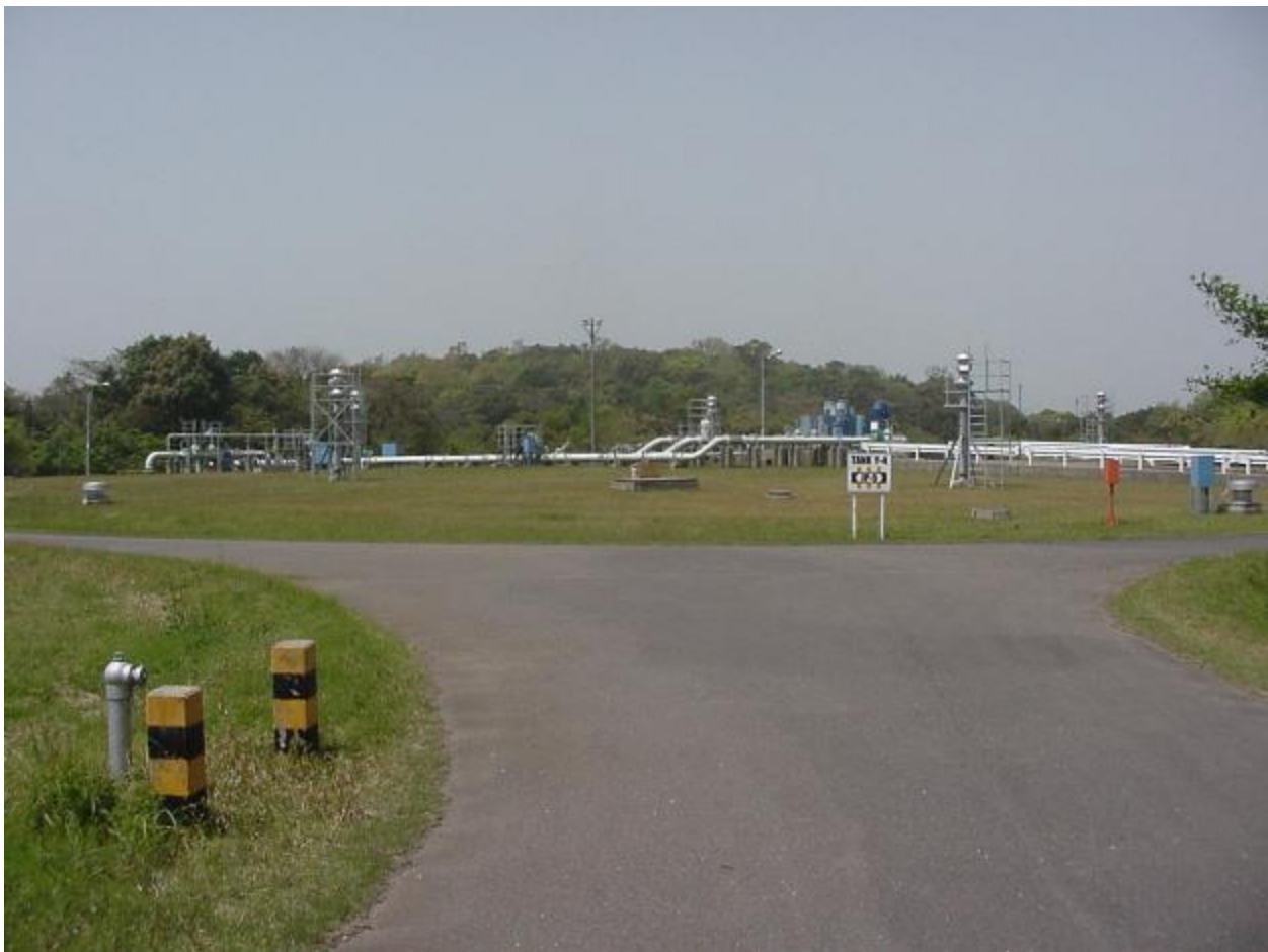
Exterior of Tank Y-4 – Tank Top
