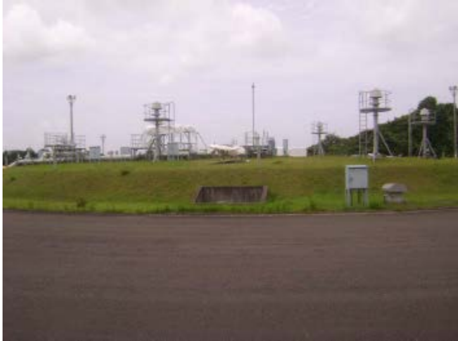
Exterior of Tank Y-8 – East Elevation
