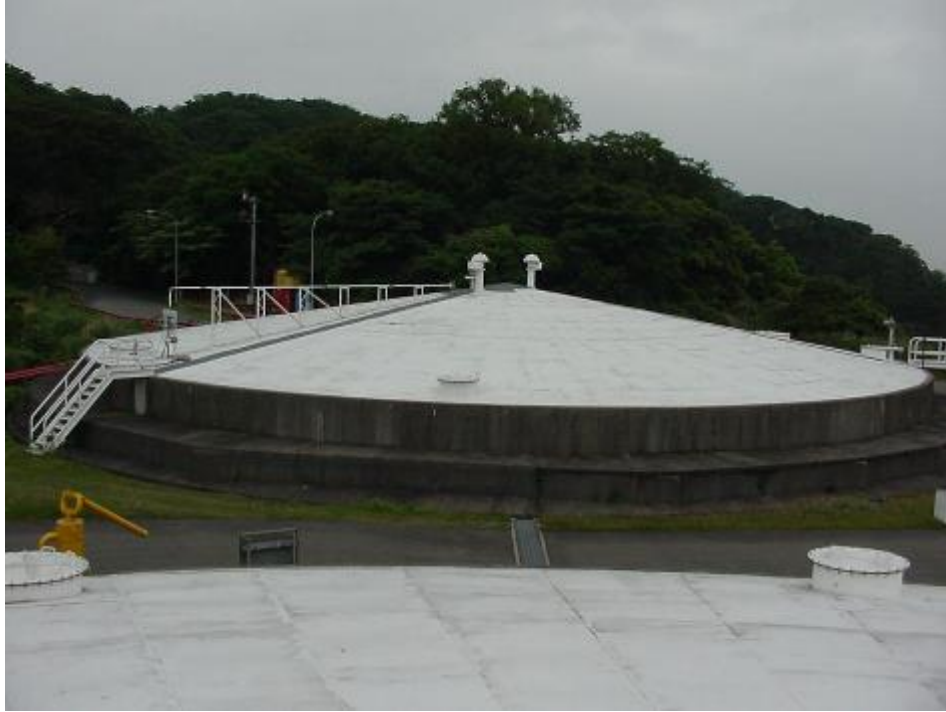
Tank 113 – Tank Top
