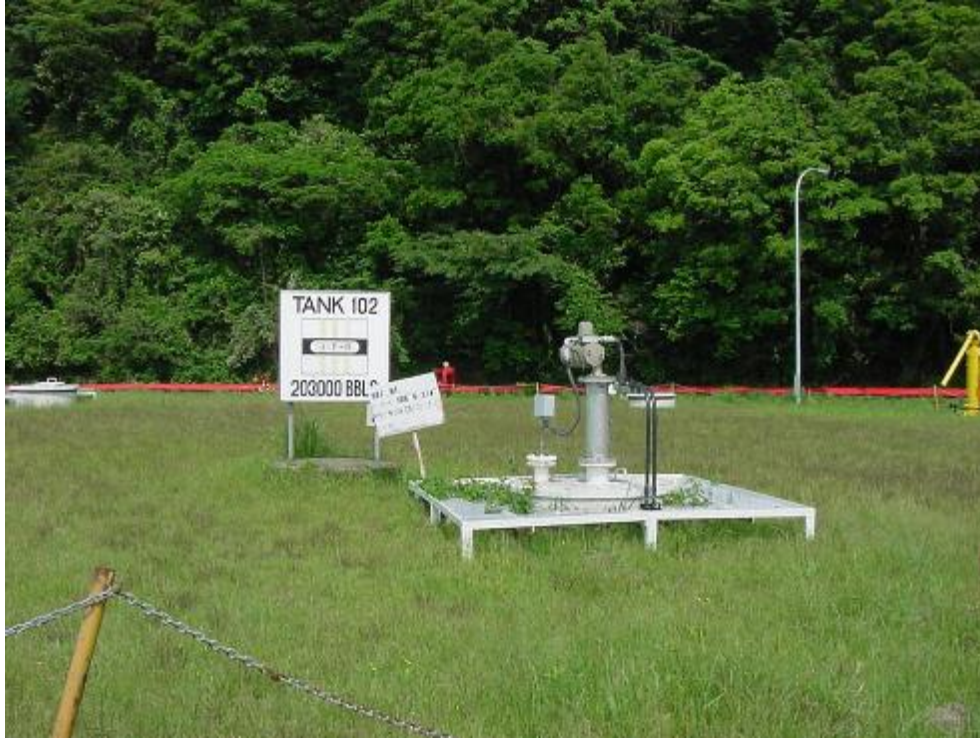
Tank 102 – Tank Top
