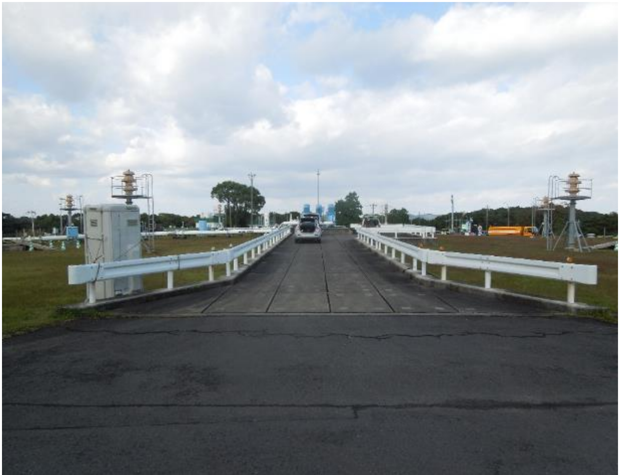
Exterior of Tank Y-7 – West Elevation
