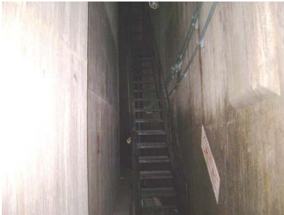
Ladder and Stair Access in Gallery Space (Typical of 4) Note: Original tank barrel is on the right side; tank shell is on left.
