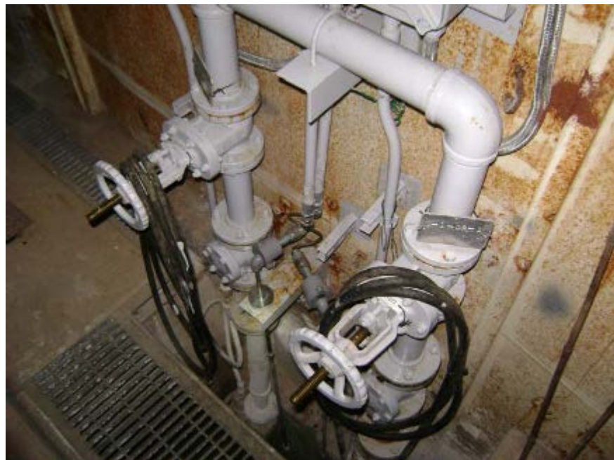
Gallery Space Sump Pump (Typical of 8)
