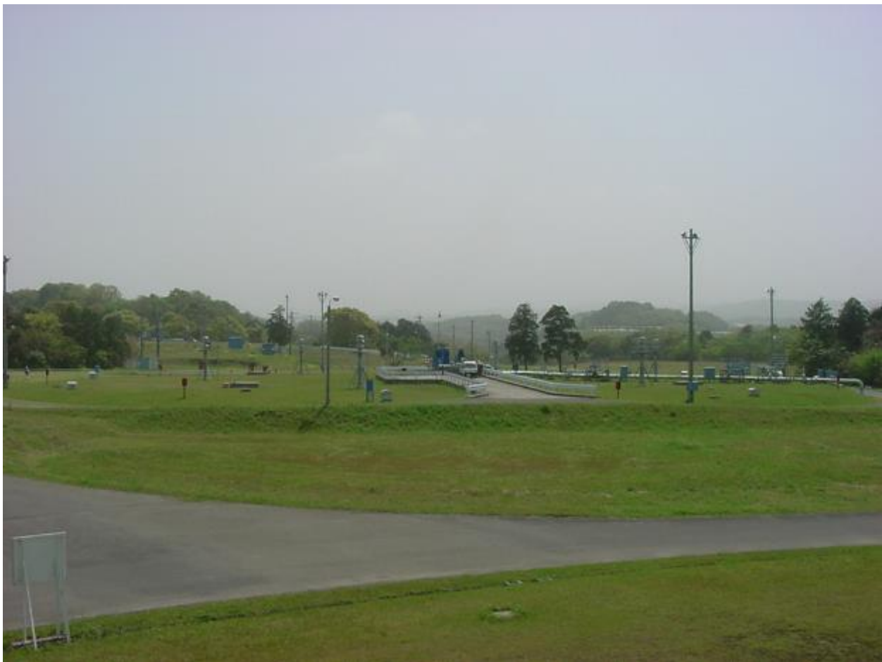
Exterior of Tank Y-6 – Tank Top
