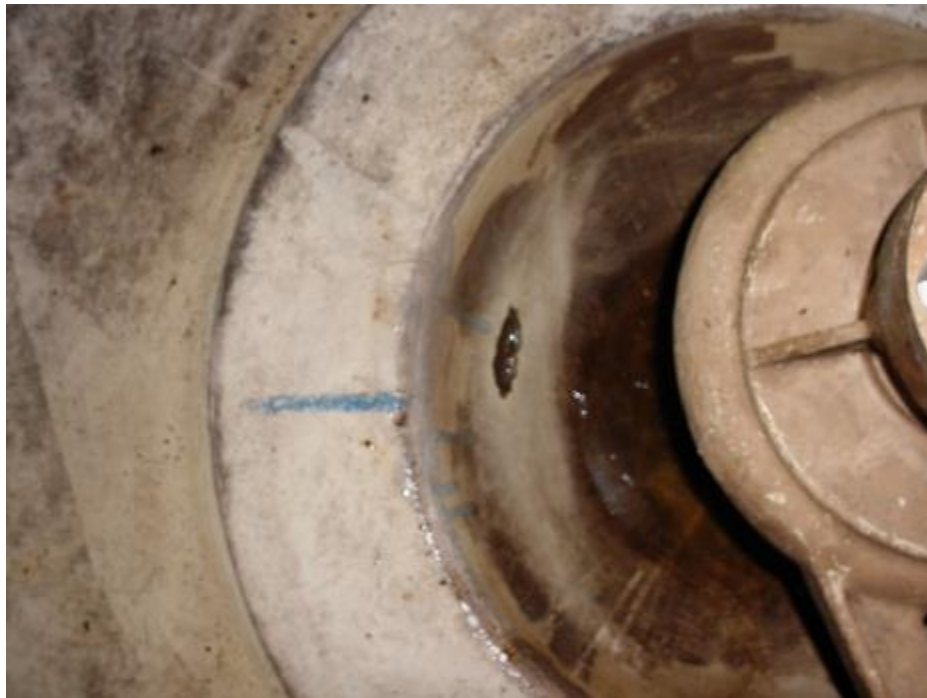
Hole in Sump
