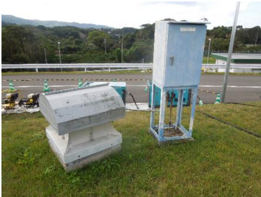
Exhaust Fan Serving to Ventilate Gallery (Typical of 8)
