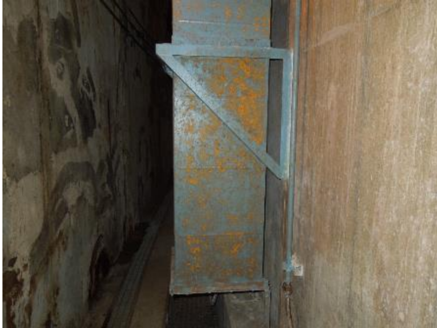
Gallery Ventilation Ductwork
