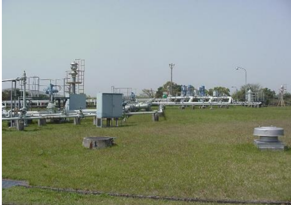
Exterior of Tank Y-2 – East Side
