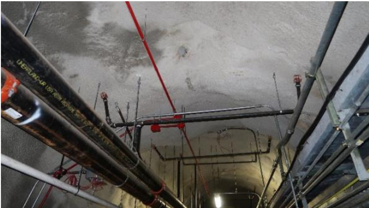
Water pipe, sprinkler heads and electrical utilities impede access
