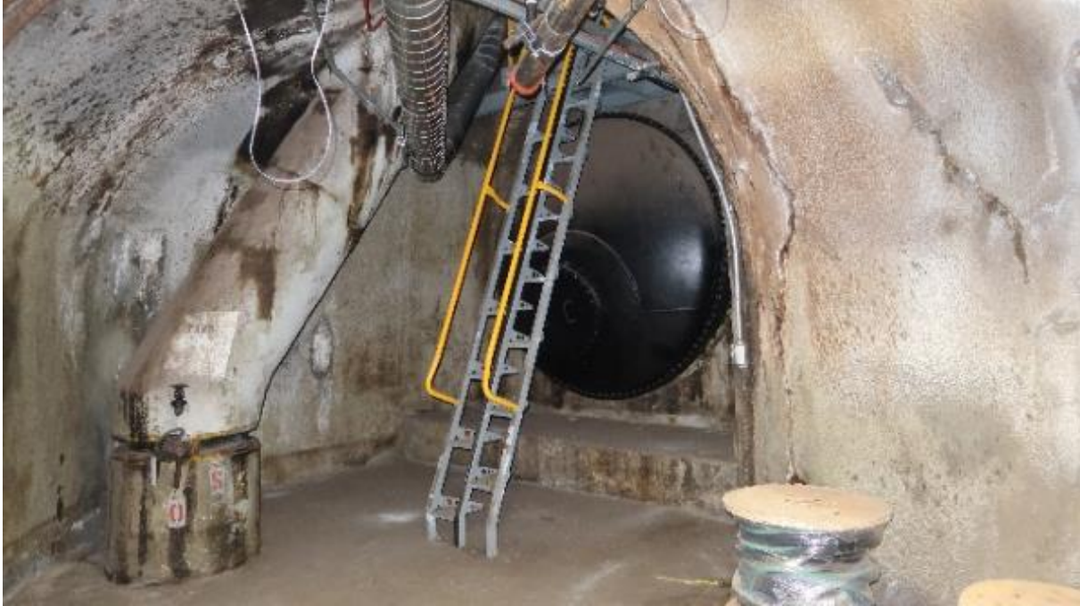
Manhole on an in-service tank. Concrete pipe at left is tank vent pipe going under the floor. Ladder provides access to the gauging gallery at the top of the tank. All materials must be loaded through manhole. Note tank ventilation pipe left of the ladder.
