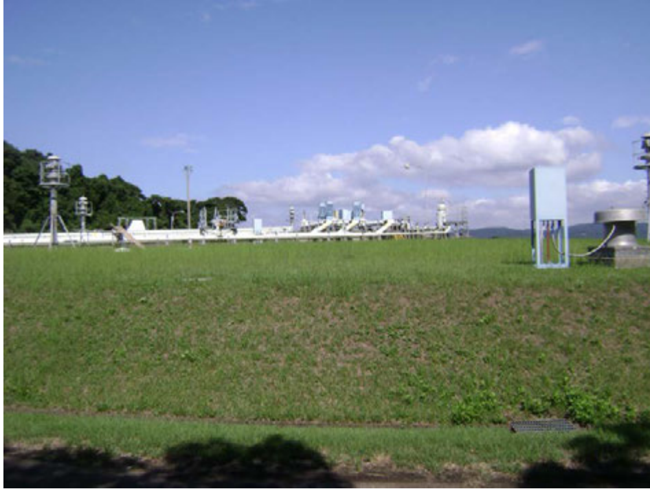
Exterior of Tank Y-3 – East Side
