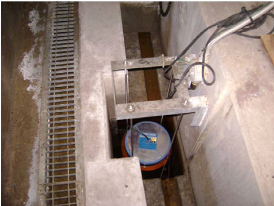
Oil Leak Detection Alarm in Gallery Space
