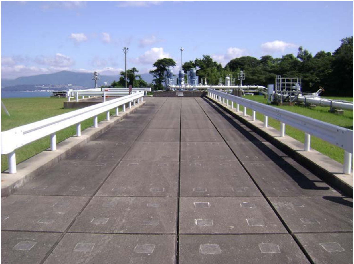
Exterior of Tank Y-3 – South Side
