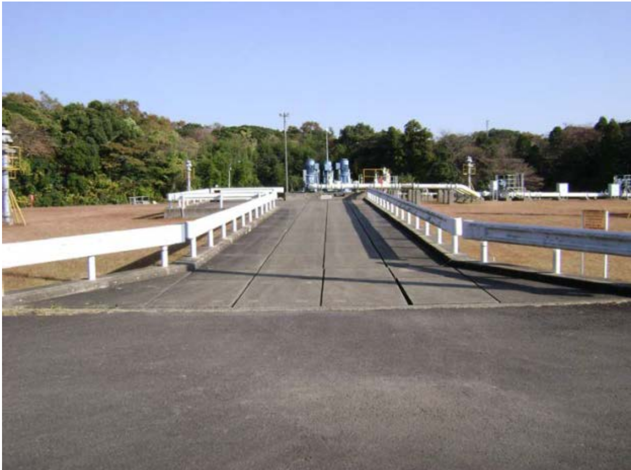
Tank Y-1 Elevation View – West Side
