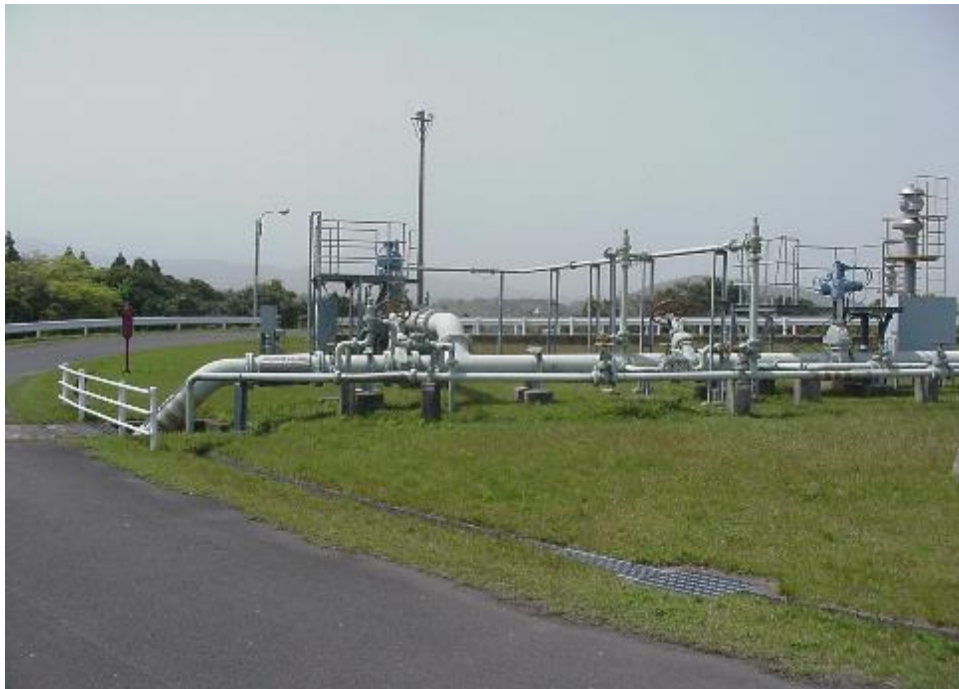
Exterior of Tank Y-2 – North Side
