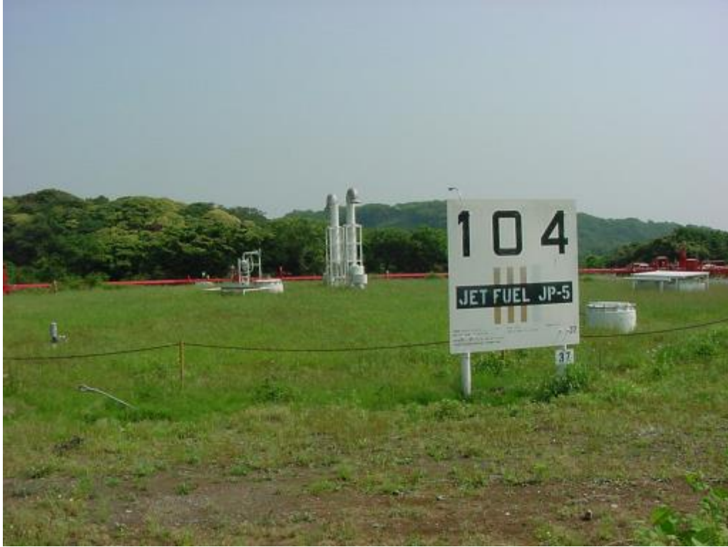
Tank 104 – Tank Top
