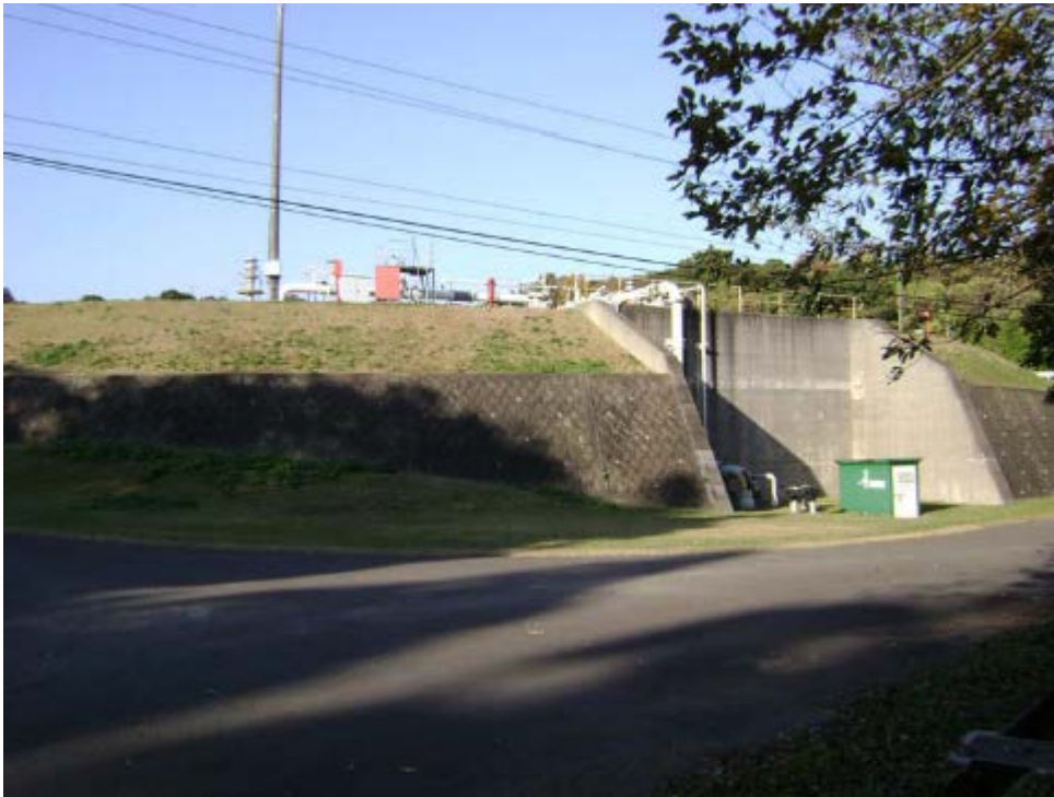
Tank Y-1 Elevation View – East Side
