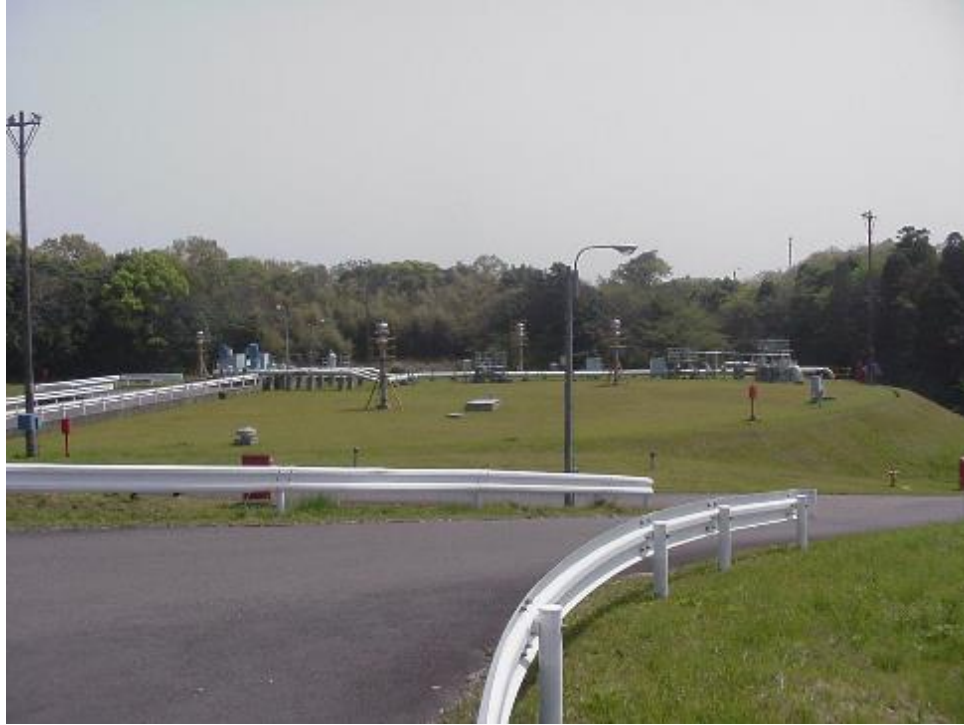
Exterior of Tank Y-1 – Tank Top
