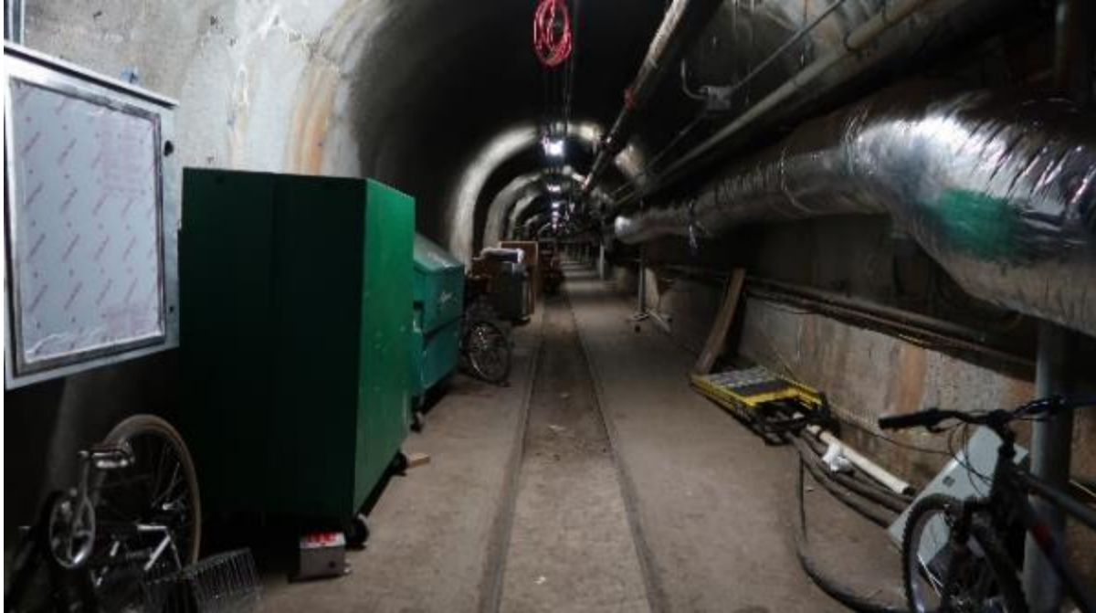
12-feet wide x 12-feet high tunnel inside Adit 4 door
