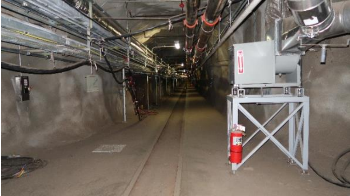
Looking down tunnel center below Tanks 1-2
