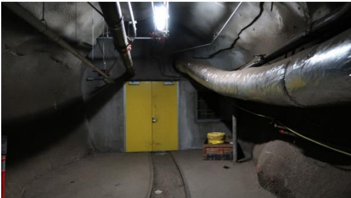
Second access door before entering tank gallery. This door and wall is required for ventilation system.
