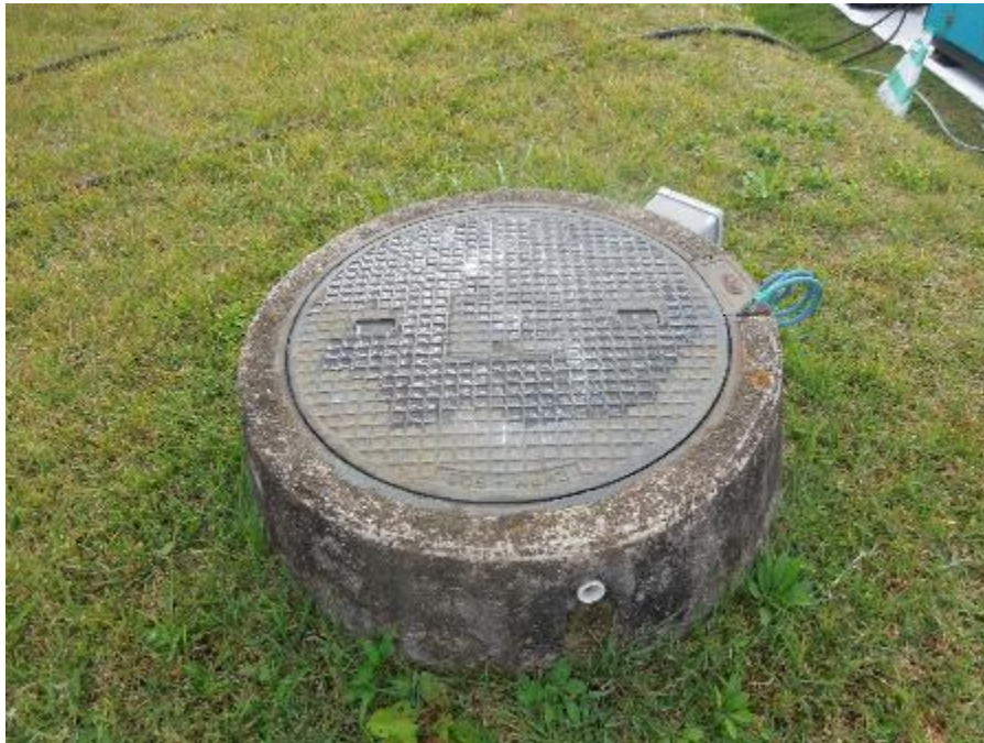
Access Manway to Gallery (Typical of 4)
