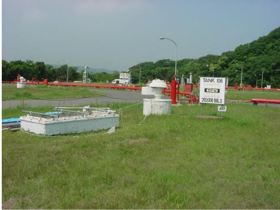
Tank 106 – Tank Top
