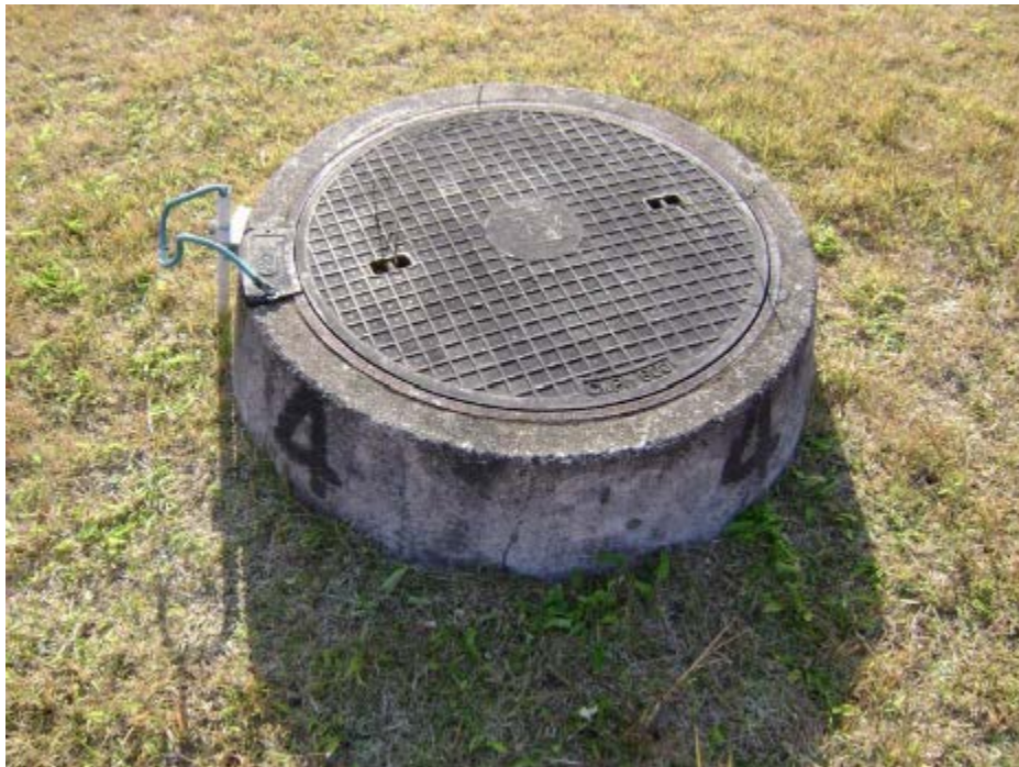
Access Manway to Gallery (Typical of 4)
