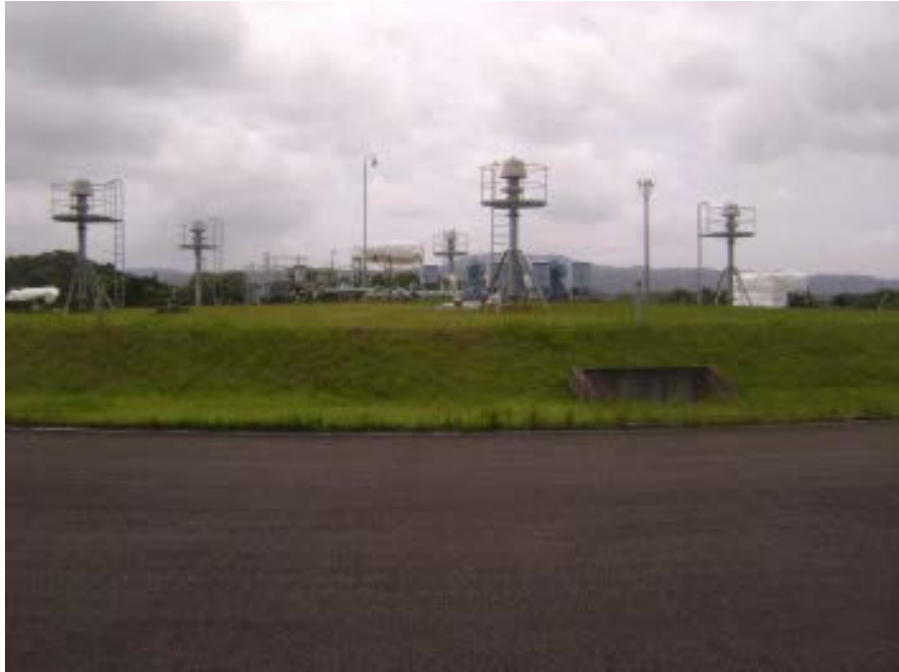
Exterior of Tank Y-8 – North Elevation
