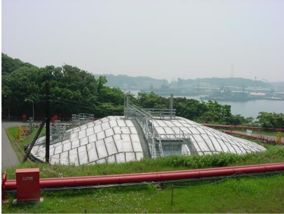
Tank 108 – Tank Top
