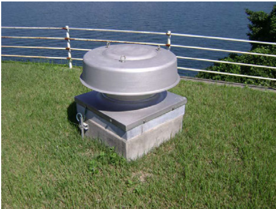
Exhaust Fan Serving to Ventilate the Gallery (Typical of 8)
