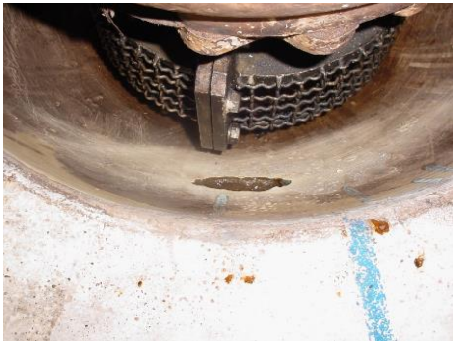
Wear Hole in Sump
