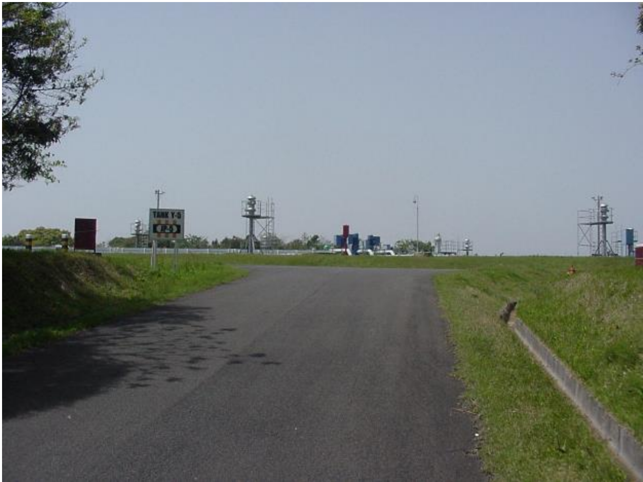
Exterior of Tank Y-5 – Tank Top
