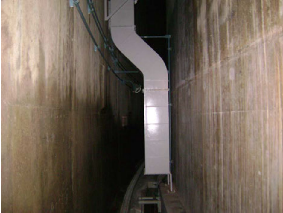
Gallery Ventilation Ductwork - Tank Barrel on Right, Gallery Exterior Wall (Cofferdam) on Left
