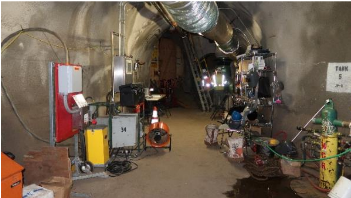
Tank 5 gallery with contractor activity
