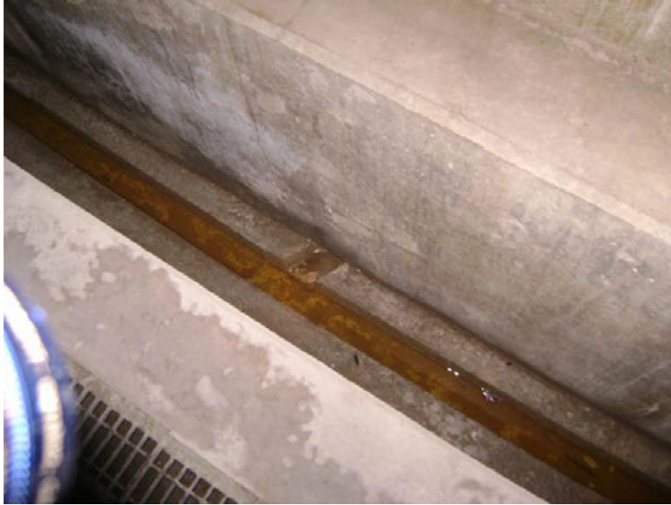
Drainage Slots Below Tank Floor Note: Slots exit to gallery trough
