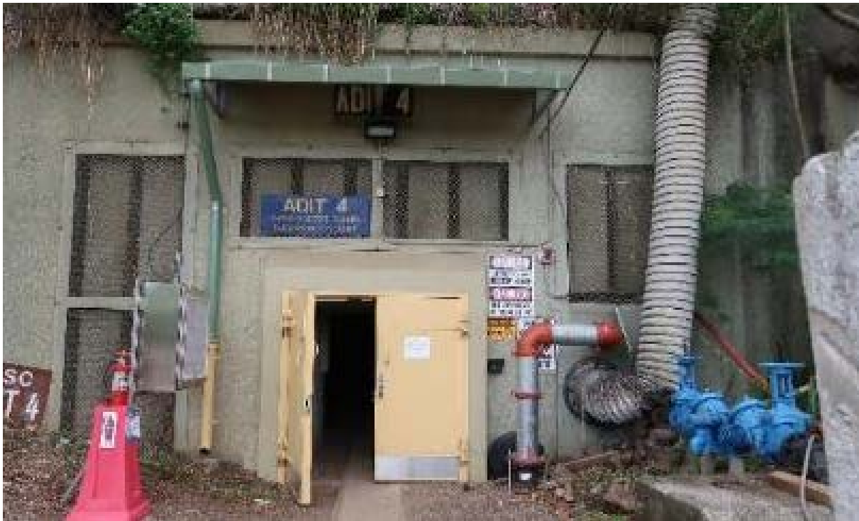
All Material must pass through this door
