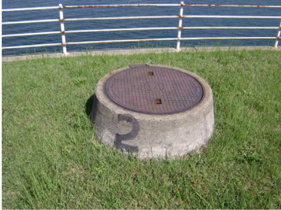
Access Manway to Gallery (Typical of 4)
