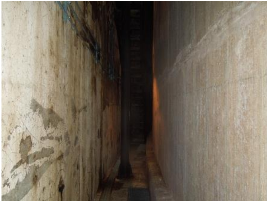
Gallery Space: Tank Barrel on Right, Gallery Exterior Wall (Cofferdam) on Left
