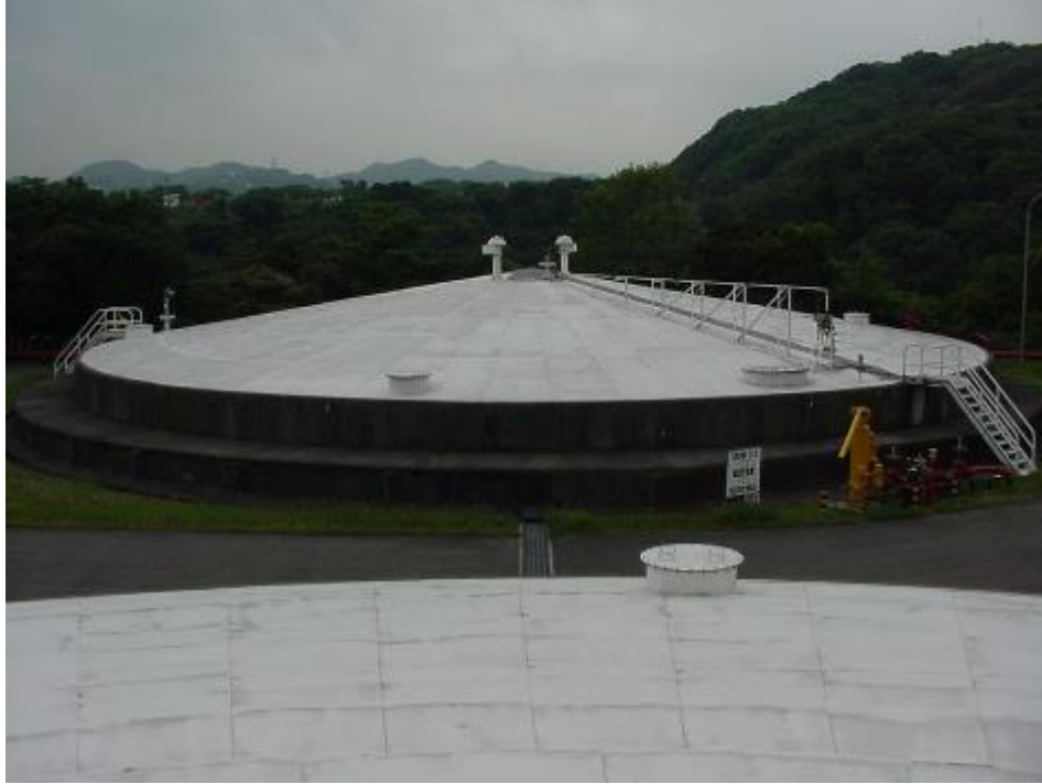
Tank 112 – Tank Top
