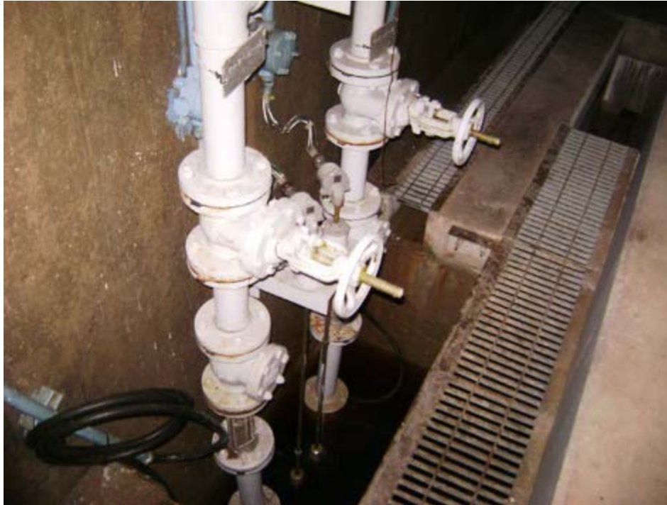
Gallery Space Sump Pump Note: This location is the gallery low point and main sump pump
