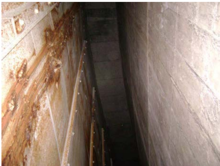
Gallery Space: Tank Barrel on Right; Gallery Exterior Wall (Cofferdam) on Left; Ceiling Above
