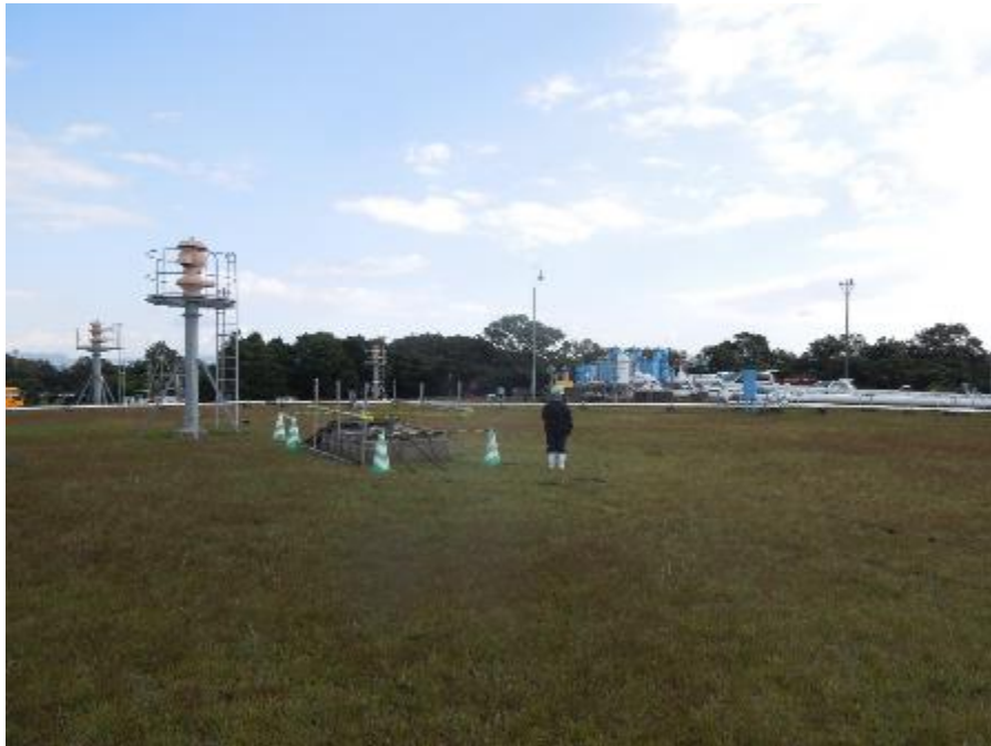
Exterior of Tank Y-7 – North Elevation
