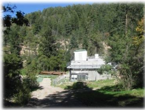
Figure A.4-1. Wastewater treatment plant
