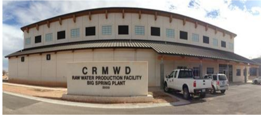
Figure A.5-1. CRMWD raw water production facility (Source: TWDB, 2015)
