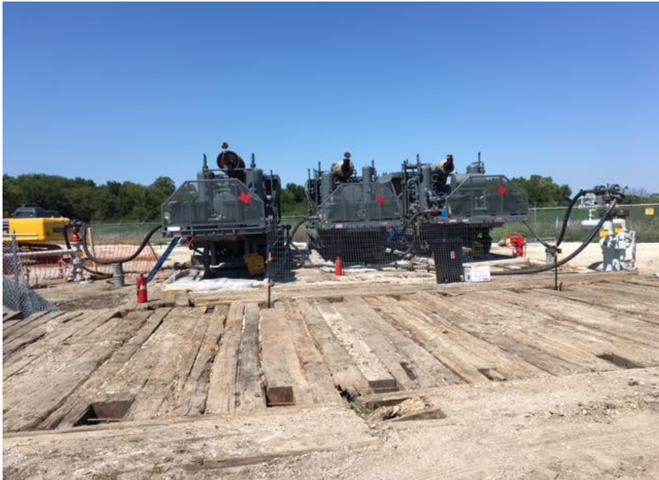
Three 300-hp compressors in parallel operation
