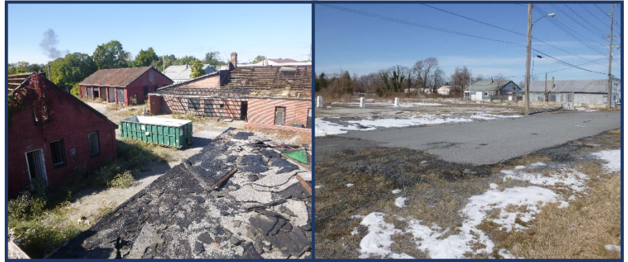
Former Chesapeake Supply before (left) and after (right) remediation. (Source: Compliance Environmental, Inc.)
