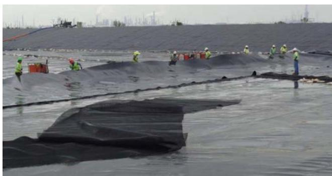
Liner being installed in base of RCRA cell at the Malone Service Company hazardous waste cleanup site, Texas. (EPA photo)
