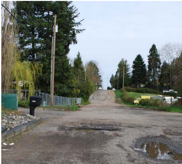
Figure 7: This unimproved section SE 89th Avenue is an example of the several streets in the Jade District. The local street network has limited connectivity to other areas of the district and includes several dead-end streets, unimproved streets, and limited bikeway connections.
