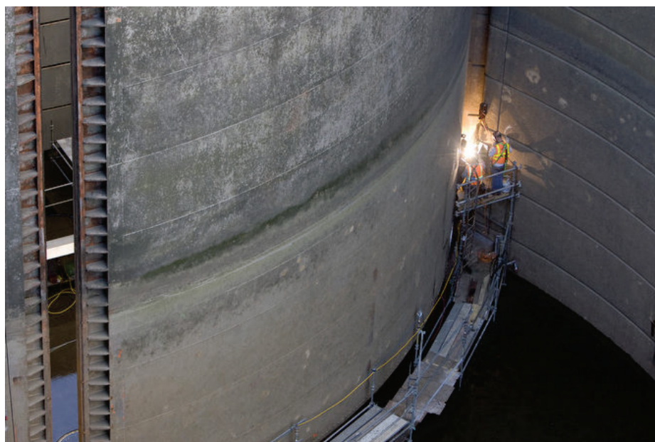
Figure 6. Repairs conducted on a lock gate at The Dalles Dam.
