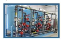
Greensand filtration water treatment plant for the removal of iron, manganese, and arsenic.
