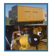
Above: 750 kW generator at Fox Ridge water treatment plant. Below: Diesel engine with starting motor for 750 kW generator
