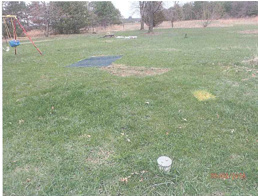
201: P5030109 Description: Septic collection field Location: SO3 Date/Time: May 3, 2018/1:09 PM
