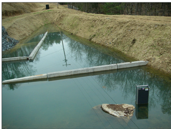
Figure 3. A limestone settling pond treats an AMD discharge.
