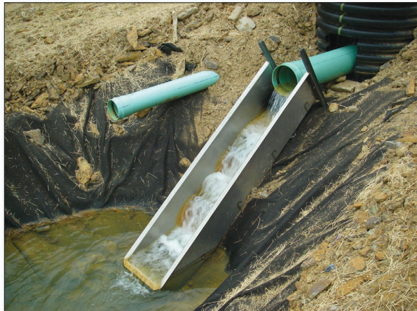
Figure 2. An aerator helps to neutralize acidity and raise pH in the Sixmile Run drainage.
