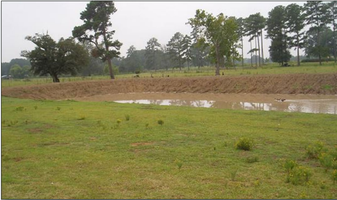
Figure 2. Water and sediment control basins were used to trap sediment and runoff from agricultural areas.
