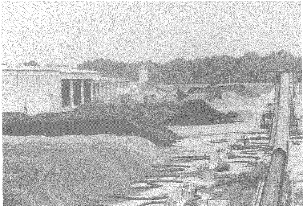
Composting can eliminate pathogens in biosolids (Columbus, Ohio).
