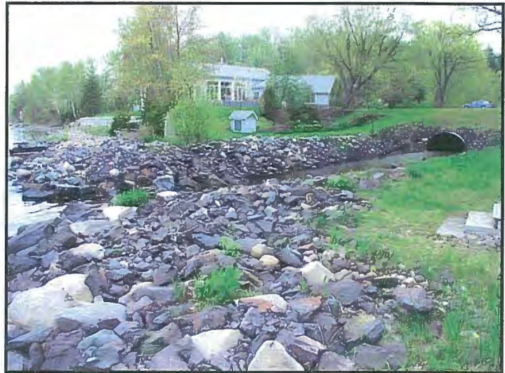
The stream crossing at Zeba Creek was remediated with a new arched culvert with a natural bottom designed for fish passage and rock armoring of the creek's outlet below the culvert which dramatically curtailed erosion.
