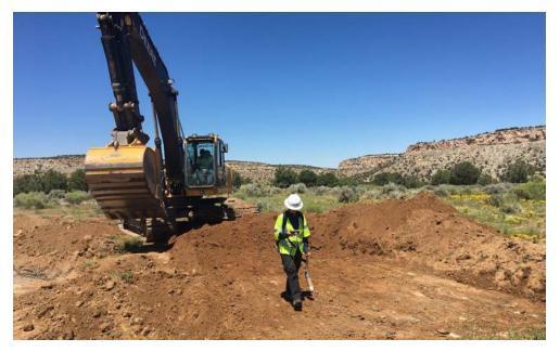
Scanning for radiation to check if the excavation is complete in this spot during the 2017 Ouivira Removal Action.
