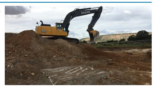
Excavating contaminated soil near a ventilation shaft during the 2017 Quivira Removal Acton. The cement cap on the ventilation shaft is in the foreground.
