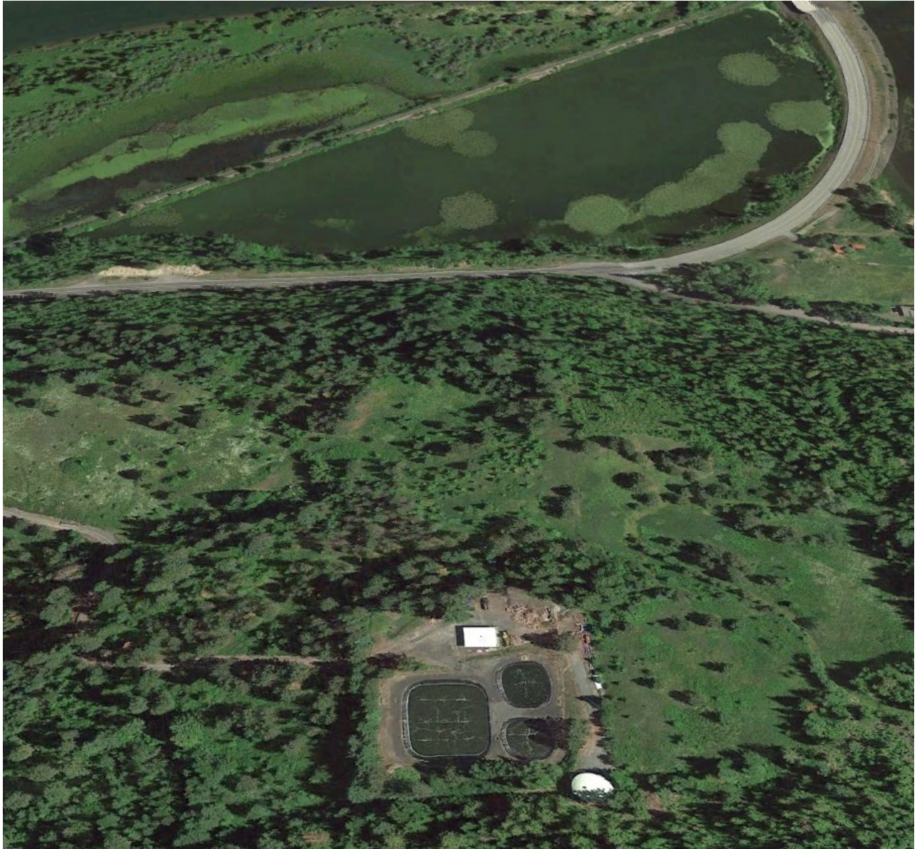
Figure 1. Harrison WWTP and Anderson Slough, Harrison, Idaho (Google Earth Pro, 6/20/17)
