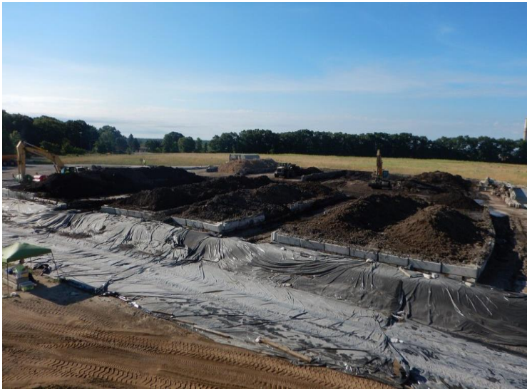
Sediment is temporarily placed at the staging area for drying (dewatering) prior to transport to a landfill for off-site disposal.
