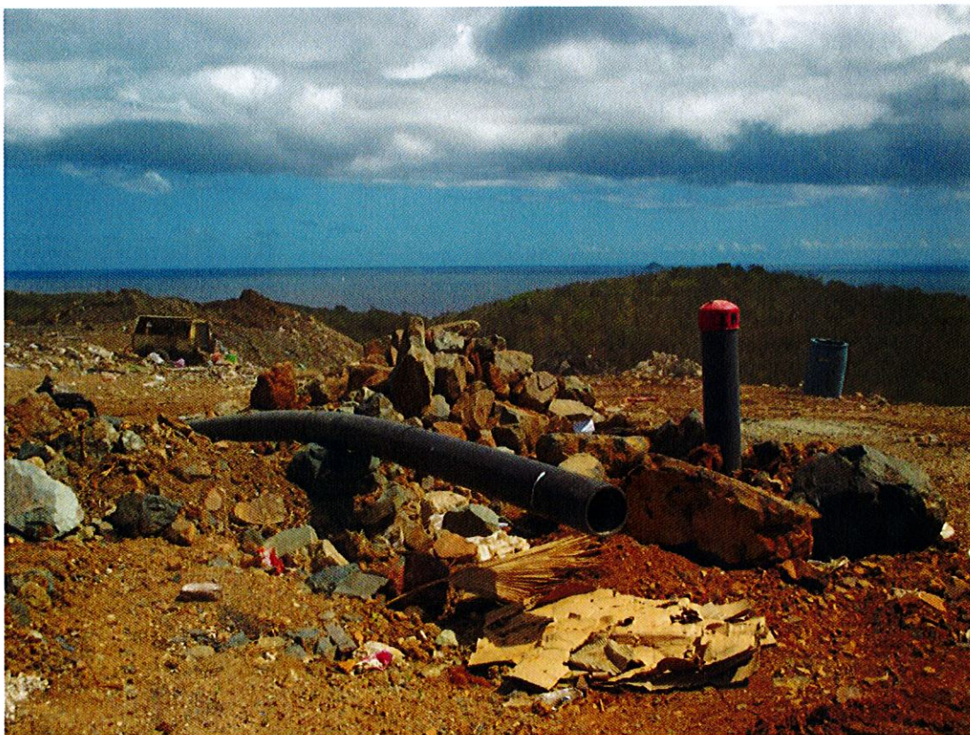
Photograph 7: Monitoring Well that has been capped – Not in use
