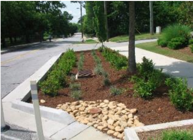
Example of a stormwater planter “bump-out” in Southeast Atlanta
