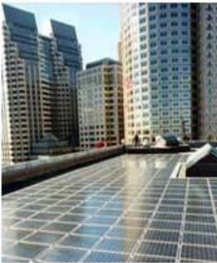
Figure 1: Solar panels (or arrays) installed on the roof of an office building..
