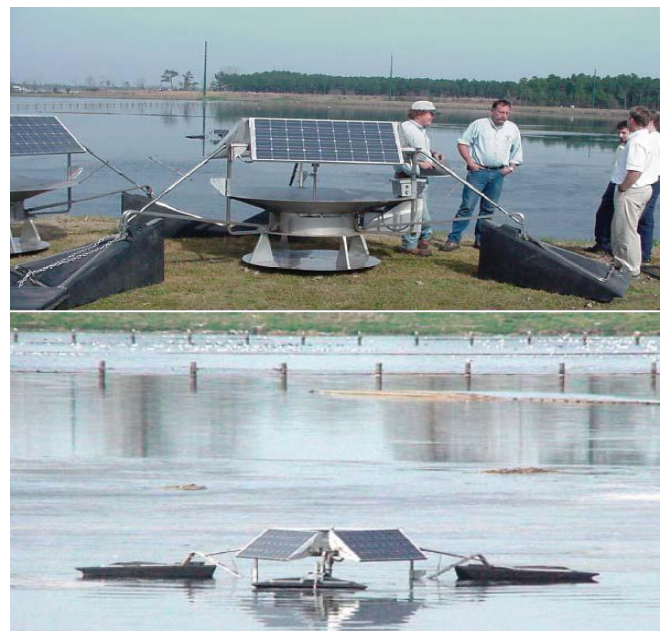
Figure 7: SolarBee® Installed in City of Myrtle Beach, South Carolina, 50-Acre Wastewater Lagoon
