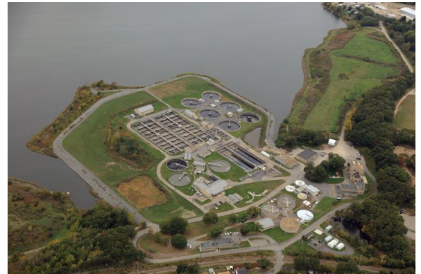
Bucklin Point Wastewater Treatment Facility
