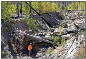
A member of the Pueblo of Santa Clara constructs a log mattress and log dam in one of the flood-eroded drainages in the firedamaged Santa Clara Creek watershed.
