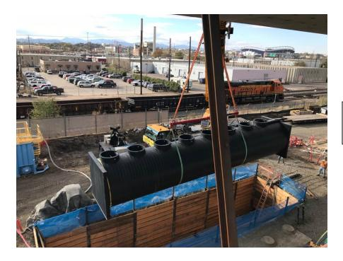
Moving Bed Biofilm Reactor placement
