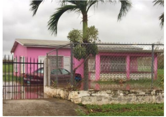
St. Croix residential flooding.
