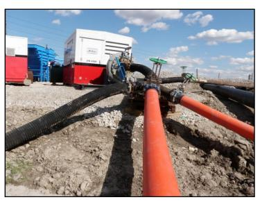
Photo 4-3. Y Connection at 10-inch Booster – Booster #1
