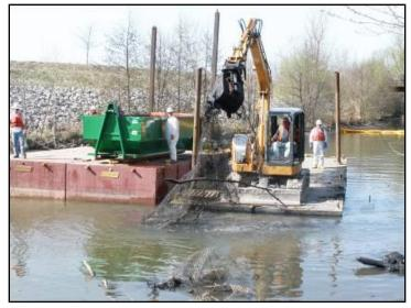
Photo 4-15. Geo-grid Removal from Ottawa River in Reach 3
