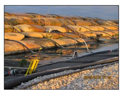
Photo 4-7. Geotubes Stacked Five High in Non-TSCA Pad
