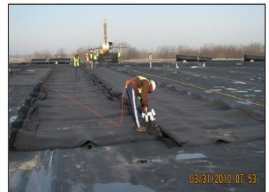
Photo 4-5. Sewing Geocomposite Layer
