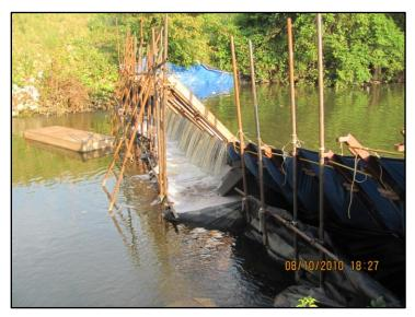
Photo 4-13. Temporary Dam Structure in Reach 4
