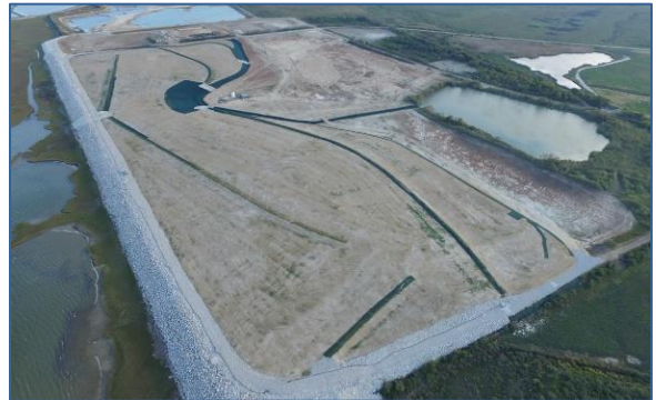
Consolidated waste cells at the Malone Services Company Superfund Site in Texas City, Texas.
