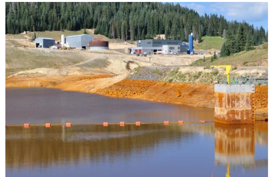
Dam impoundment and upgradient water treatment plant at the Summitville Mine site in the San Juan Mountains of Colorado.
