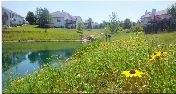
Figure 2. Native plants were planted along the shoreline of a basin in the Huntsdale Subdivision.
