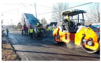
**Photo #2:** View during installation of the asphalt intermediate base coat for Forsythe Street
