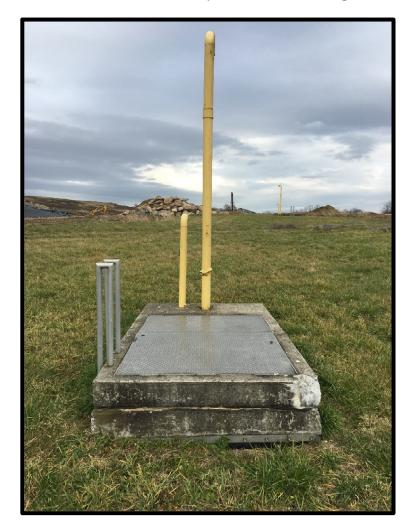
Picture 6: Passive Ventilation System at Mountain Top Landfill
