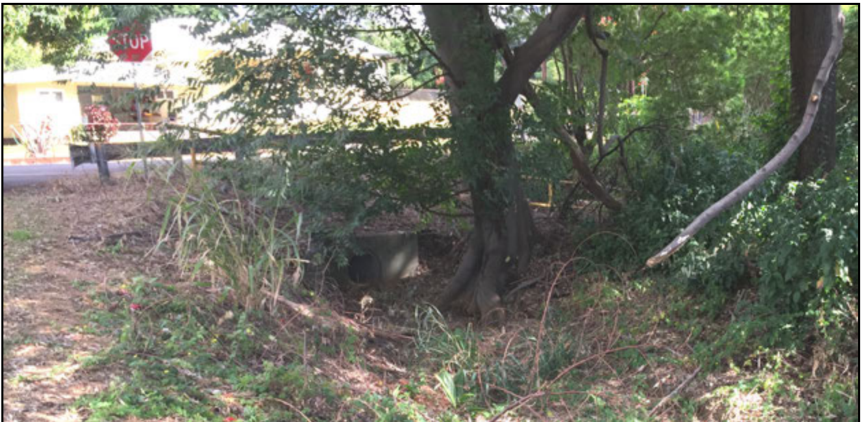
Figure 31. Photo of the culvert located at the Huapala Street and Ilima Street intersection; view to northeast
