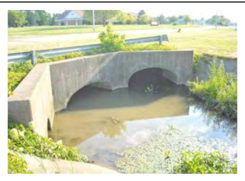
Figure 3-19 Three large culverts are located immediately upstream of the Amlosch Ditch sampling location (AD-1). The center culvert transmits upstream flow beneath Dustin Road.
