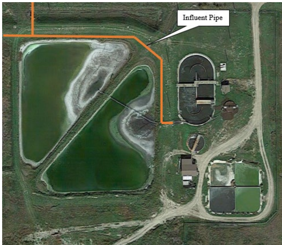
Figure 4. Aerial view of WWTF
