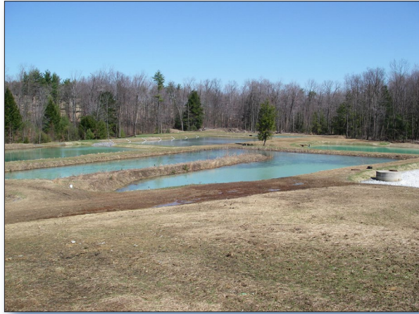
Figure 2. A passive treatment system installed at one of the four priority sites.
