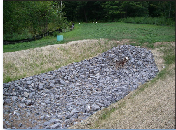
Figure 3. A buried anoxic limestone drain empties into a limestone channel.
