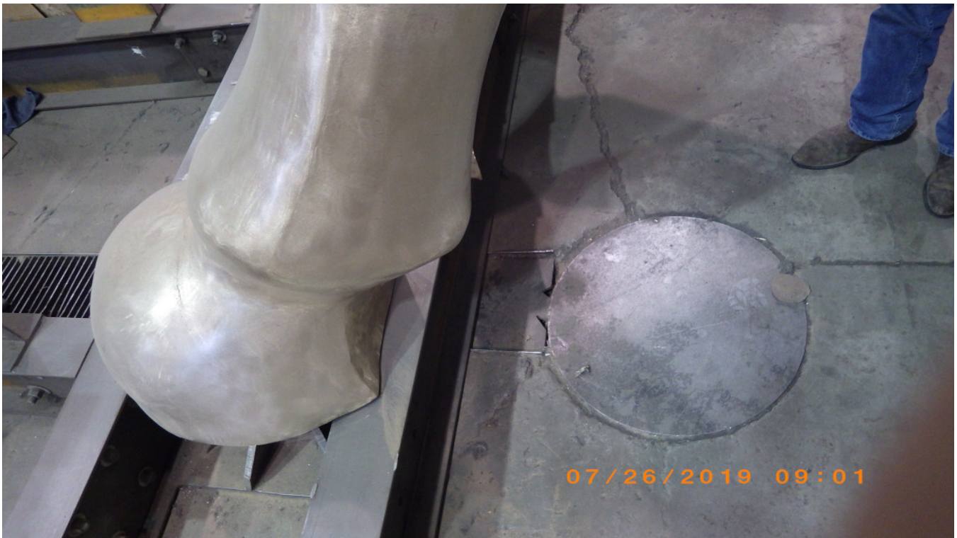
Figure 5 - Monument Building Floor Sump
