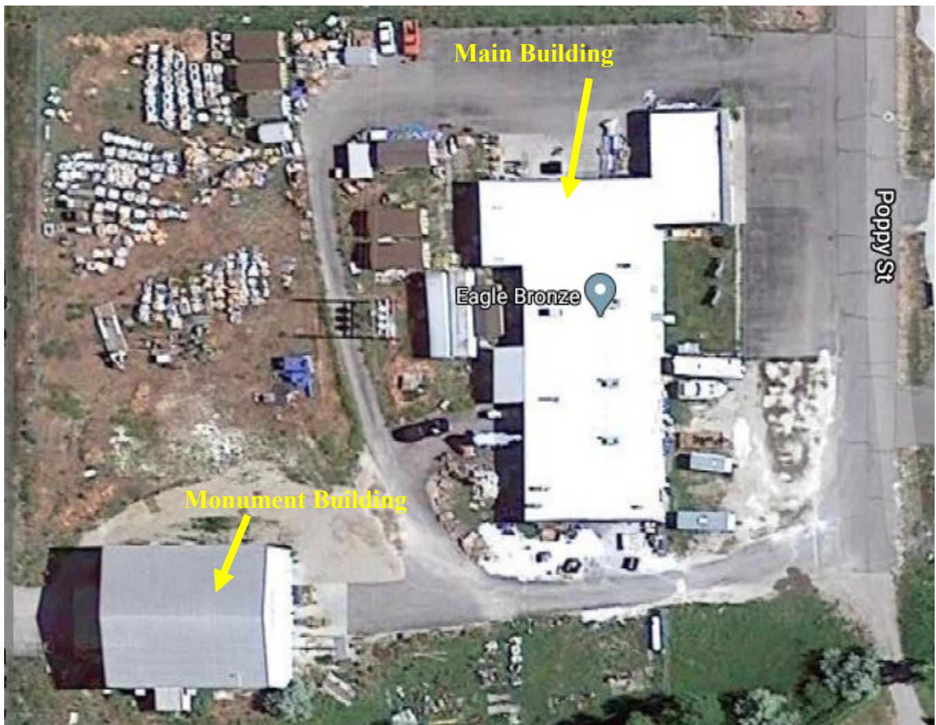
Figure 1 - Eagle Bronze Facility - Google Earth View
