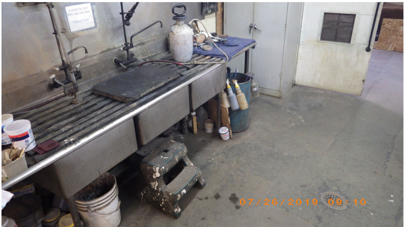
Figure 2 - Main Building Patina Sink and Floor Drain
