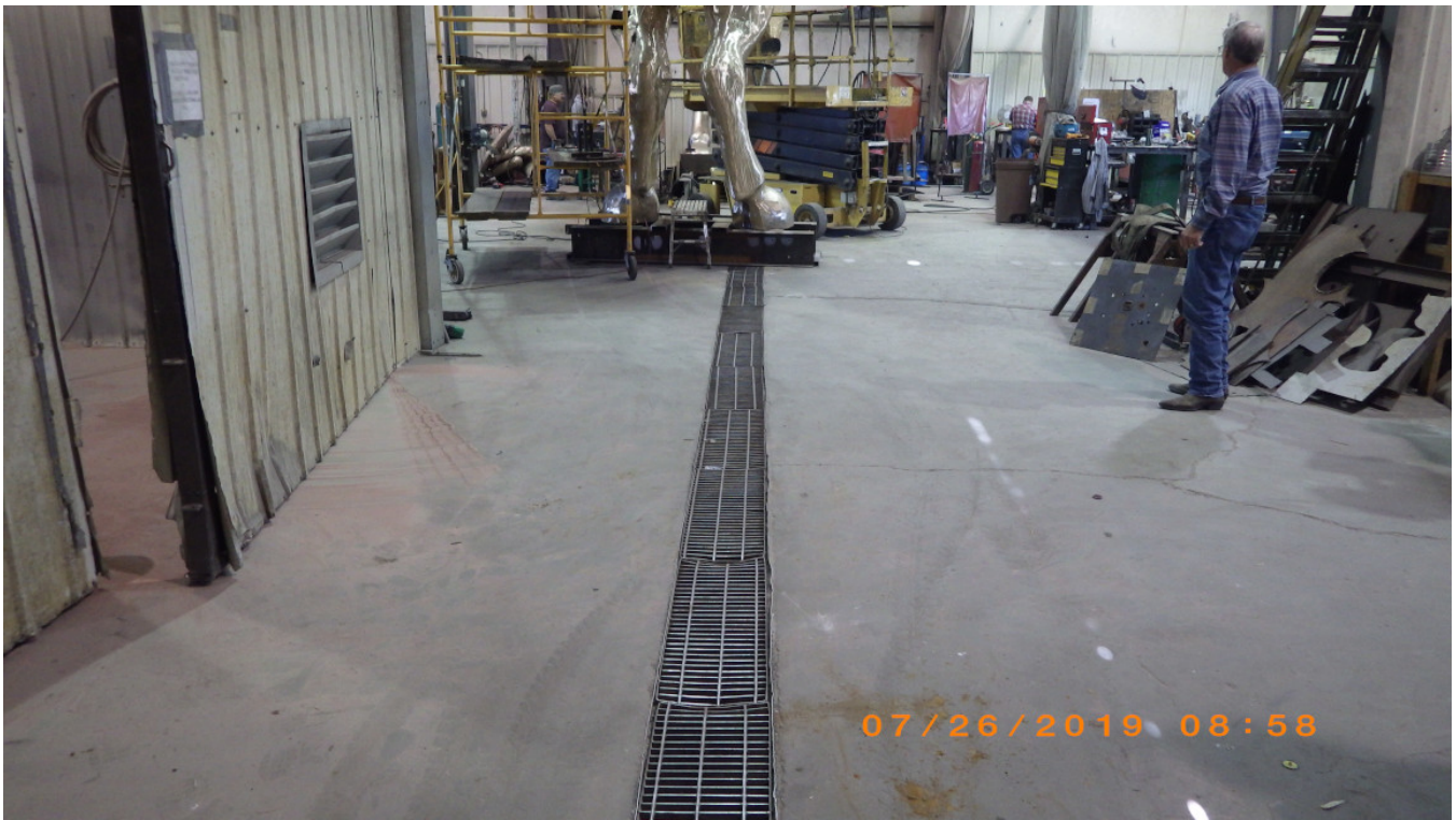
Figure 4 - Monument Building Trench Drain
