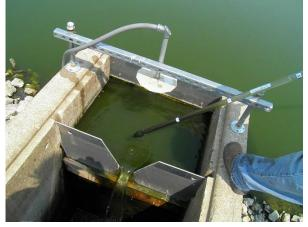
Figure 4. Algae and sludge Can Both Leave the Pond System to Affect BOD
