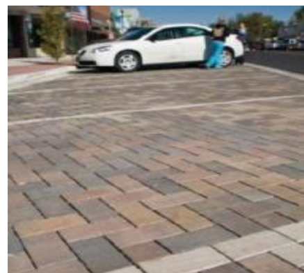
Figure 7: Permeable pavement. (Source: Pima County and City of Tucson. Low Impact Development and Green Infrastructure Guidance Manual. March 2015.)
