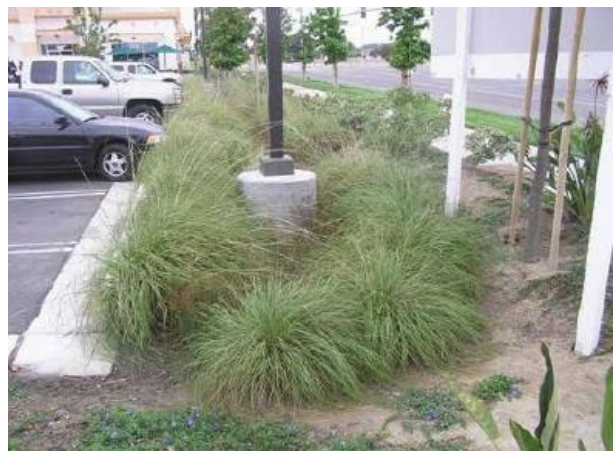
Figure 4: A bioretention system at a parking lot. (Source: Pima County and City of Tucson. Low Impact Development and Green Infrastructure Guidance Manual. March 2015.)
