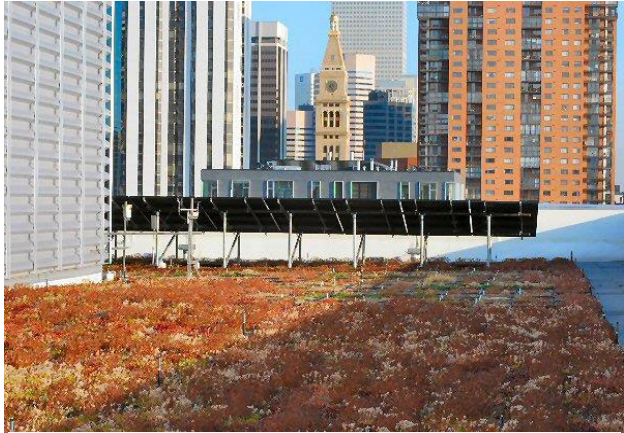
Figure 8: A green roof in Denver, Colorado. (Lee, J., & Fisher, C. (2016). Arid green infrastructure for water control and conservation. State of the Science and Research Need for Arid/Semi-arid Regions. Environmental Protection Agency. )
