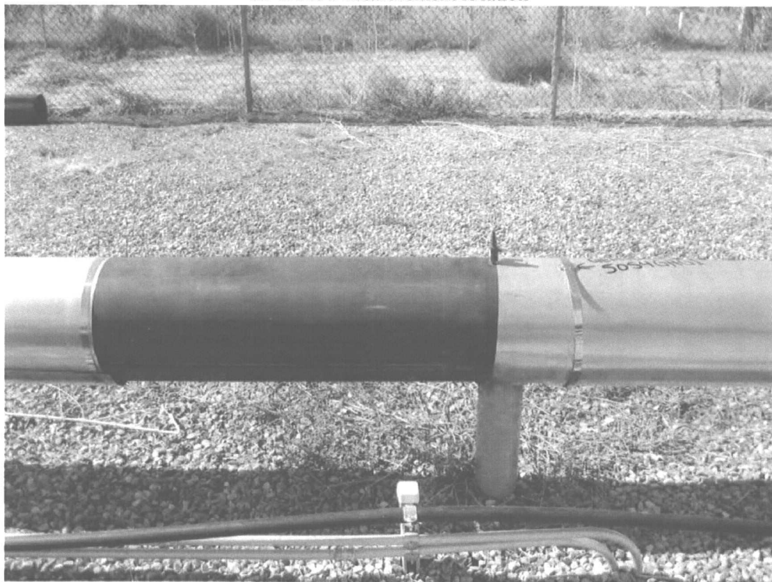
Chestnut Landfill - Gas sampling port
