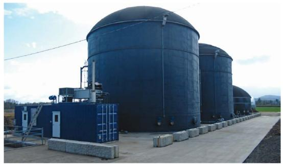
Figure 2-2. Photograph of an anaerobic digester facility (a patented sequential-batch system).<sup>2</sup>
