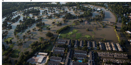
An aerial view of the flooding caused by Hurricane Harvey in Houston on August 31, 2017. (U.S. Department of Defense photo)
