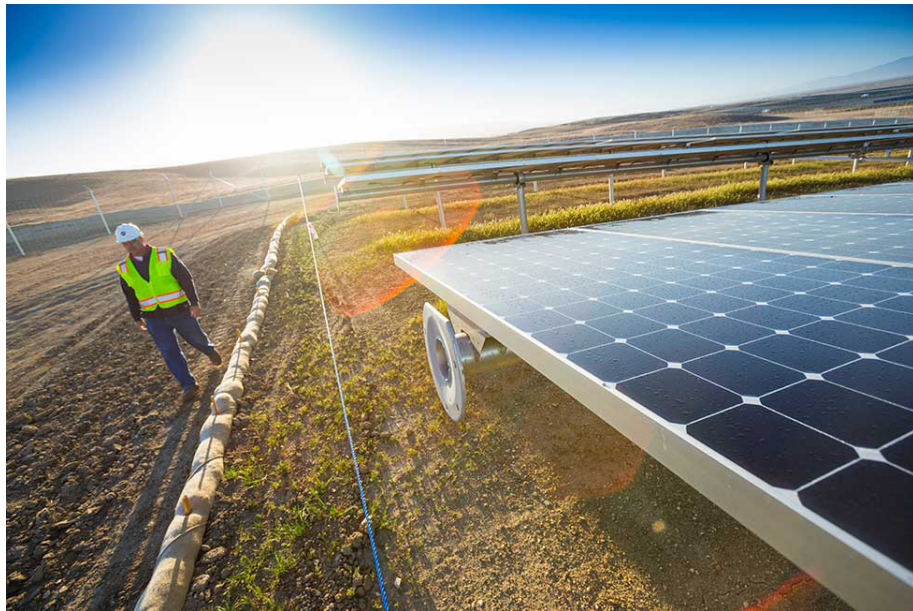
Worker checking solar panels in California.
