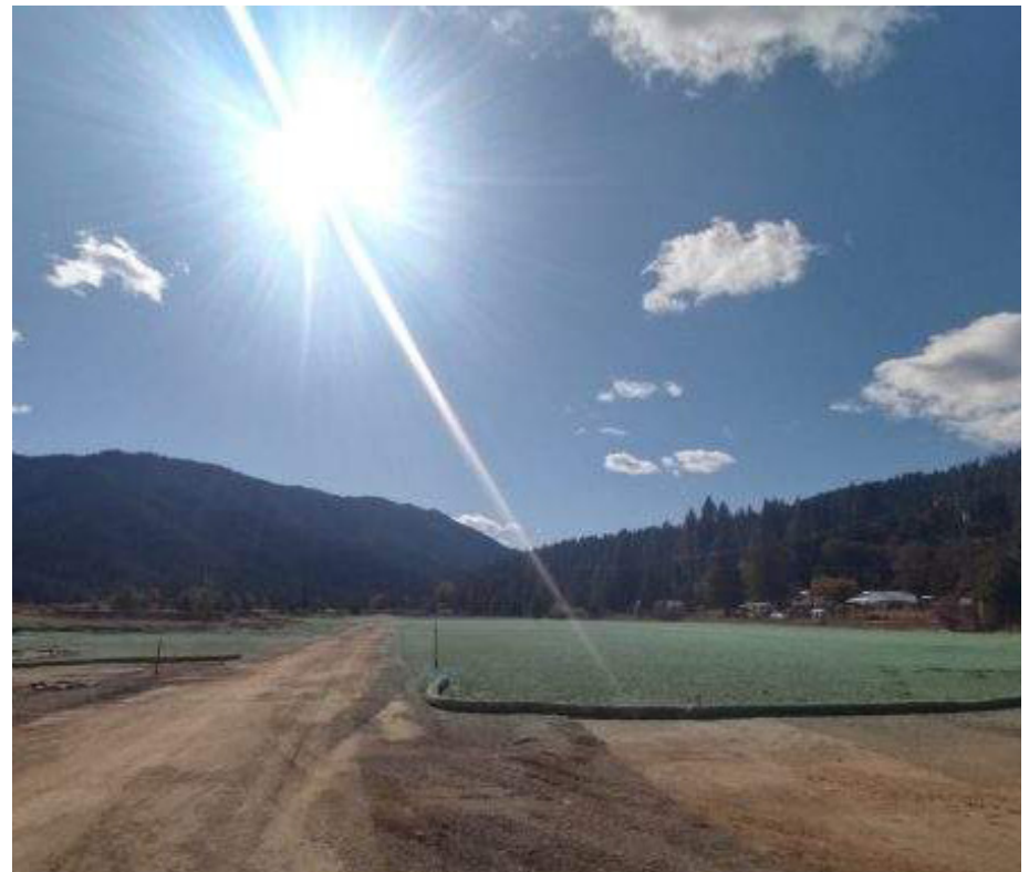
Hydromulch (green) in place to winterize the site after the end of 2019 operating season.
