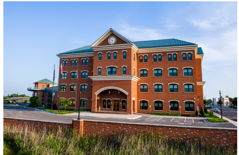
The new academic center for APUS, on the 1.8-acre site of the former Veiner Metal Salvage Yard.
