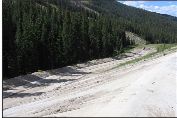
Figure 2. A snow slide BMP was constructed along I-70.
