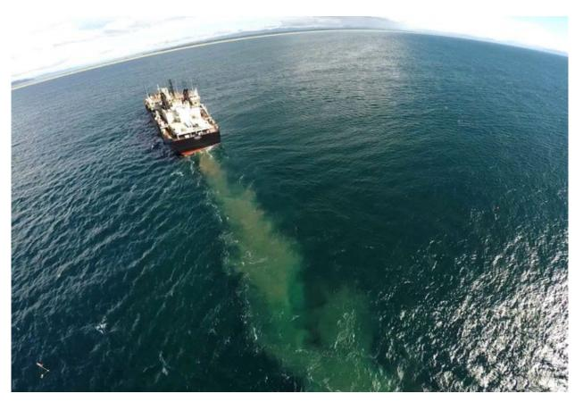
Figure 25. Aerial view of the Essayons during nearshore thin-layer sand placement operations near the mouth of the Columbia River. The disposal vessel moves forward slowly with hull doors only partially opened, so that sand is spread thinly in long, narrow tracks. The ship's propellers help to further disburse the sand.
