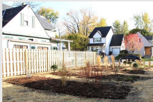
The Hulda Avenue site in Cleveland's Woodland Hills neighborhood includes rain gardens, planting beds, a fence and artisan concrete paving.
