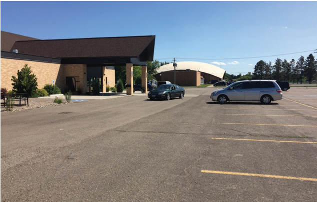
Figure 23: Current condition of the Epworth United Methodist Church parking lot.
