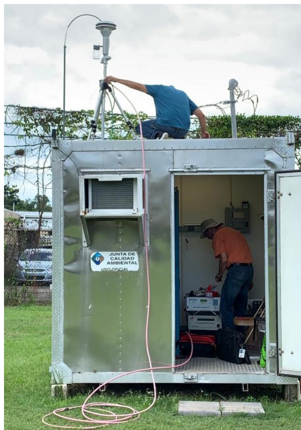
Inspecting an air monitoring station in Puerto Rico to ensure proper operations after Hurricanes Maria and Irma.
