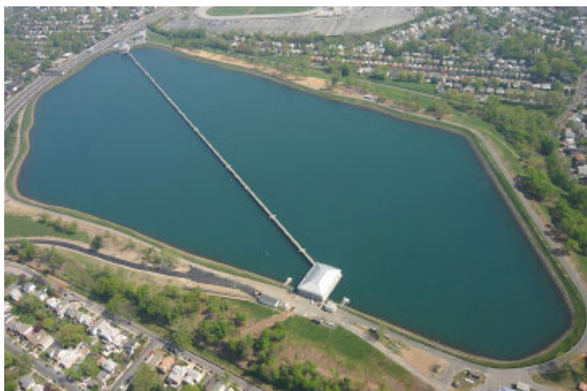
Hillview Reservoir, in Yonkers, New York, which is part of New York City's public water system.
