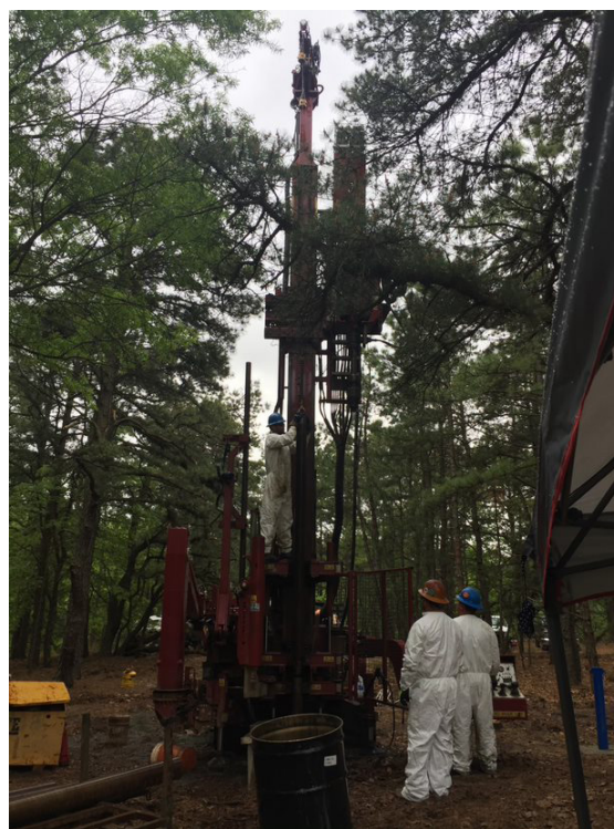
Installation of a groundwater monitoring well at the Sherwin-Williams Superfund site. Data from this well will be used to delineate the extent of contamination when designing remedial action.
