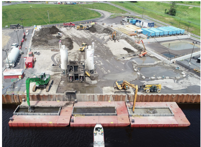
Grasse River Superfund site in Massena, NY.
