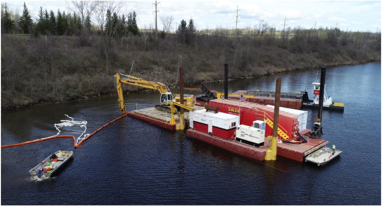
Dredging at the Grasse River Superfund Site in Massena, NY.
