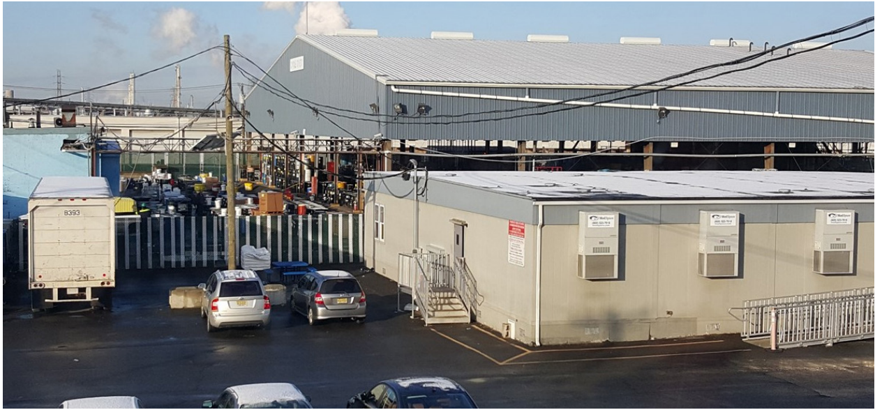
The Cycle Chem facility in Elizabeth, NJ.
