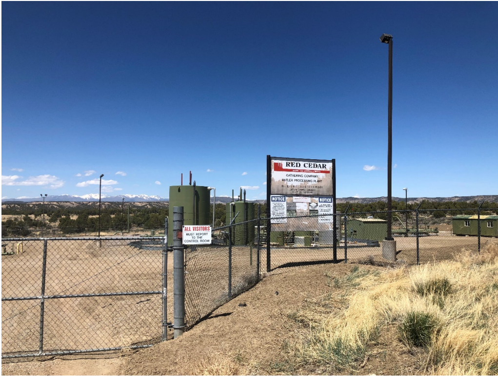
Photo 1. Entrance to Antler facility, view north.
