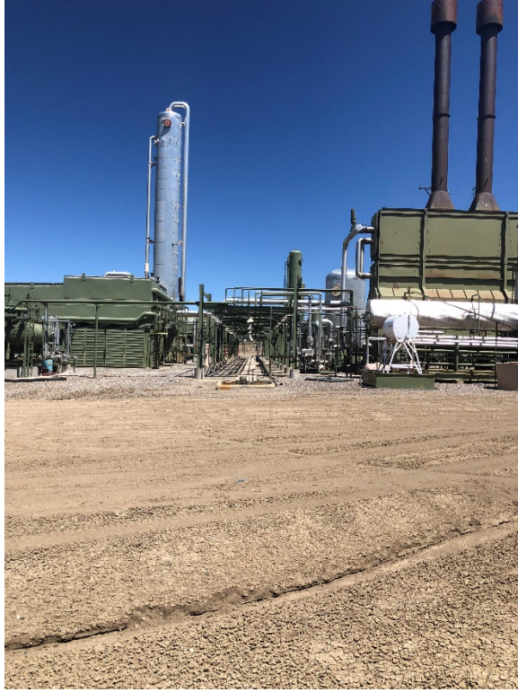
Photo 5. View east of existing equipment from west facility boundary.
