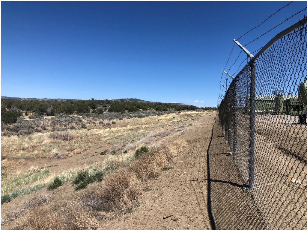
Photo 4. View east along north facility boundary.
